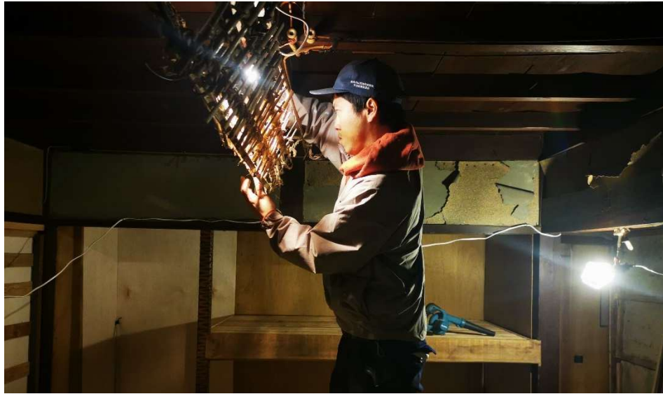
Figure 6.14. Salvaged bamboo lattice from demolished walls repurposed into lamp shade. Photo by author, December 15, 2021.
