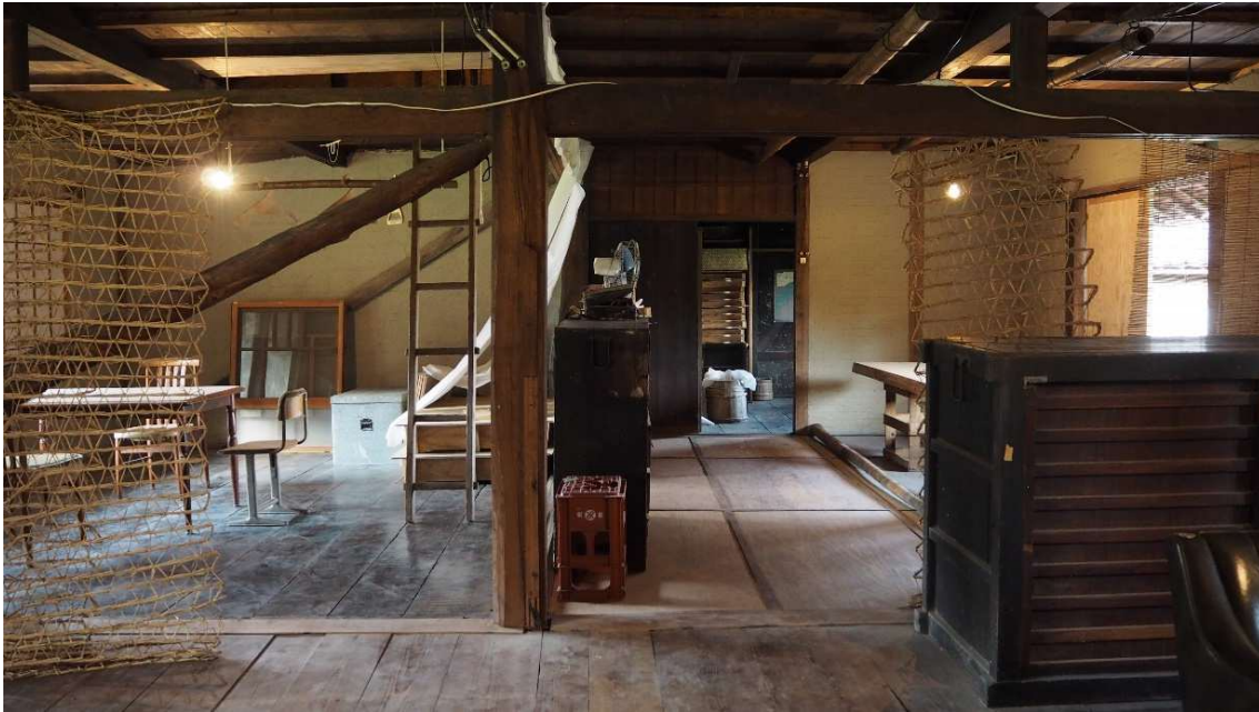
Figure 7.2. Second floor of the akiya renovated by students over the years showing newly plastered walls. Photo by author, May 3, 2019.
