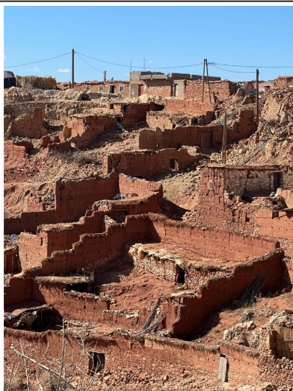
Figure 1 Rural village of Tafeghaghte in Al-Haouz Region. The earthquake heavily damaged the built environment, raising pressing concerns about rebuilding processes. Source: Keio SFC Koblabs, March 2024.
