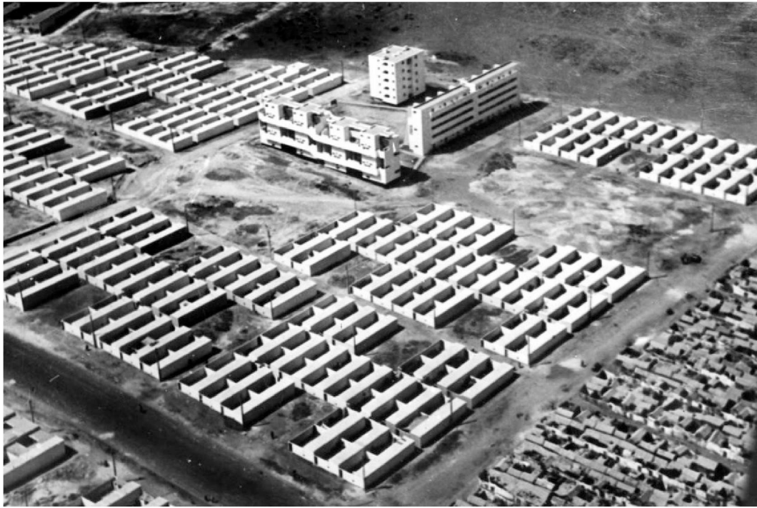
Figure 5 Carrières centrales in Casablanca. Construction of the low-rise 8x8m grids and high-rise residential buildings, including Nid d'Abeille. Source: Michel Écochard Archive, courtesy of Aga Khan Documentation Center, MIT Libraries (AKDC@MIT), 1948.
