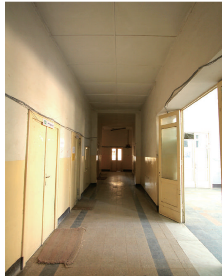
[11] A Corridor with Panel Ceiling, photo by Shimizu, N., 2015
