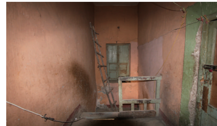
[10] A Stair Room (Upper Floor, Building-A), photo by Shimizu, N., 2018
