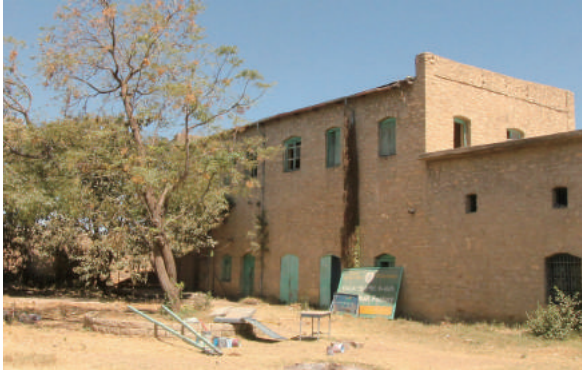
Fig.4-119 External appearance of Liquor Factory from the courtyard, photo by author.
