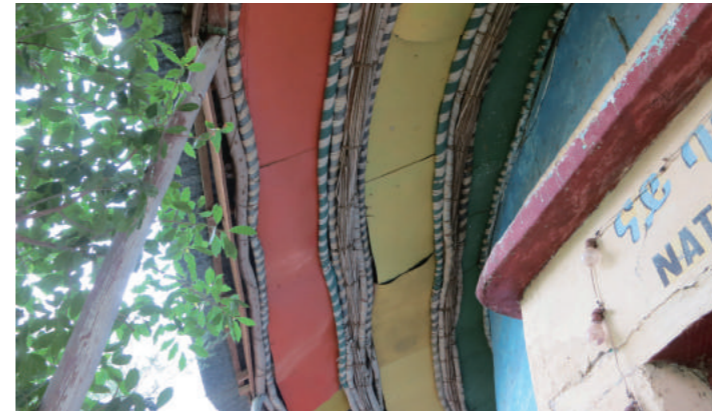
[10] Original Thatched Roof Covered with Corrugated Metal Sheet, photo by Shimizu, N., 2012
