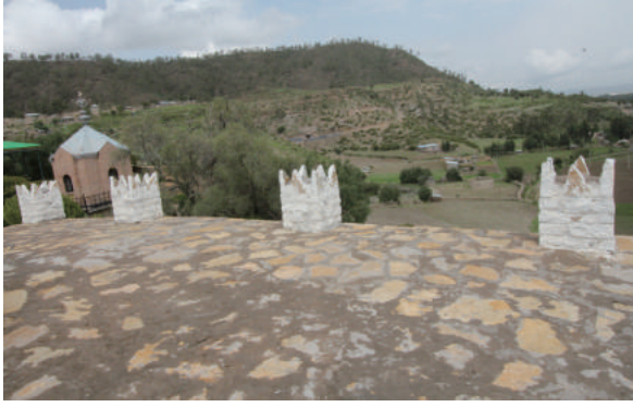
Fig.2-119 Current roof covered by stones and coronal shaped parapets, Mika'el Church in Feleg Da'iro, photo by author.
