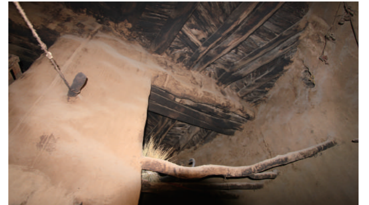
[5] A Central Masonry Pillar and A Built-in Rack, photo by Shimizu, N., 2015
