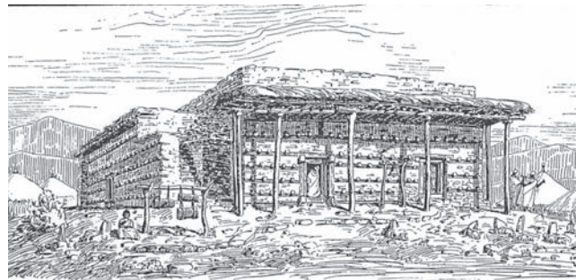
Fig.2-54 External appearance of Īnda Maryam Church in Asmara, now demolished, from Littmann et al. (1913) .
