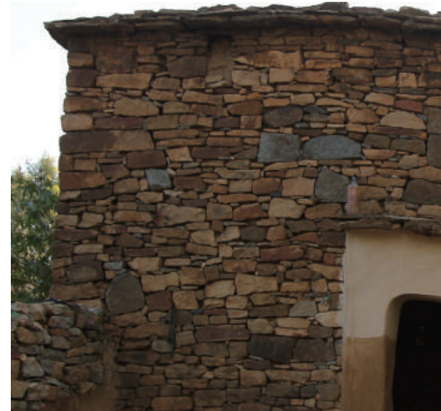
Fig.3-58 Corner part of hidmo house, photo by author .
