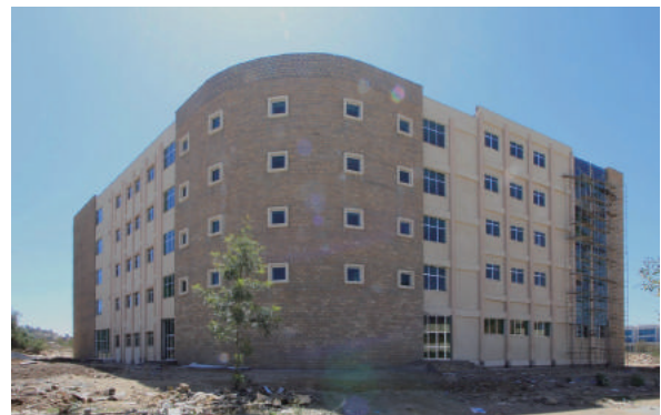
Fig.6 A building of IPHC in Mekelle University Arid Campus, photo by Aoshima, K.
