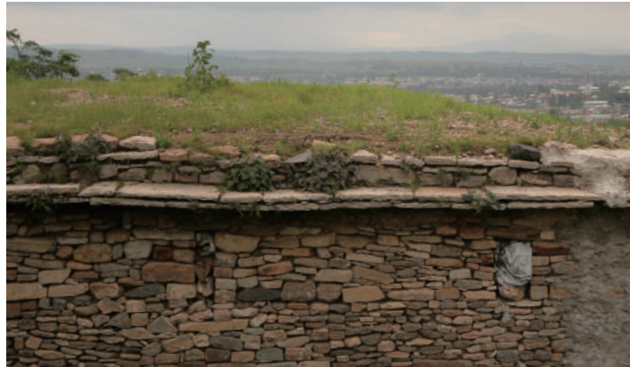
[3] Detail of Hidmo Roof, photo by Higuchi, R., 2010
