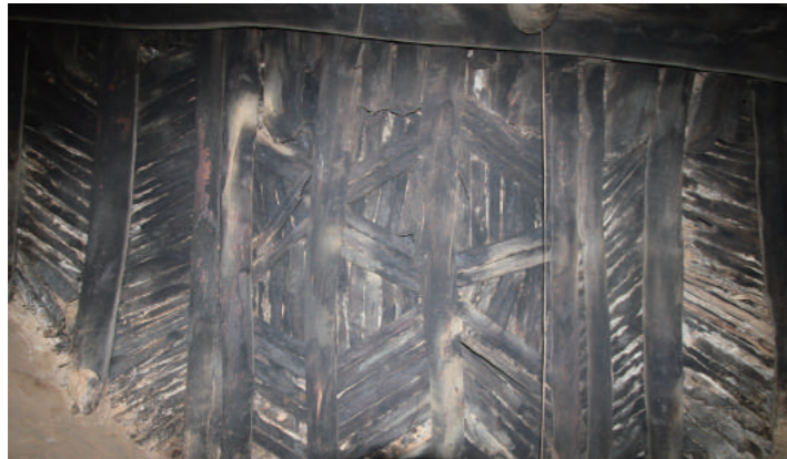
[5] Detail of Hidmo Ceiling, photo by Shimizu, N., 2015
