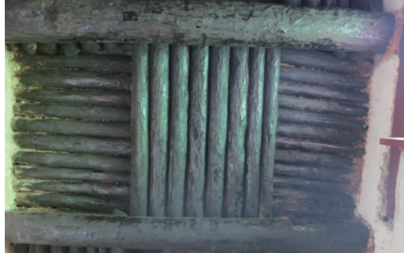
Fig.4-38 More rigid timber structure of the ground floor, Former Residence of Emperor Yohannis IV (Building-B), photo by author.
