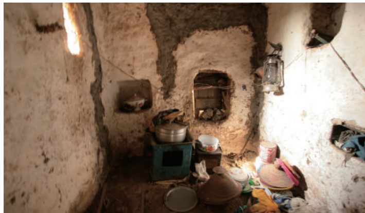
[7] Appearance of Debri (Upper Floor), photo by Higuchi, R., 2010
