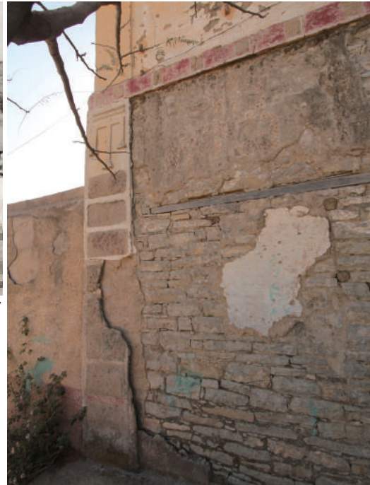
Fig.4-146 A wall of Building-A of Old Hospital Quarter, photo by author.
