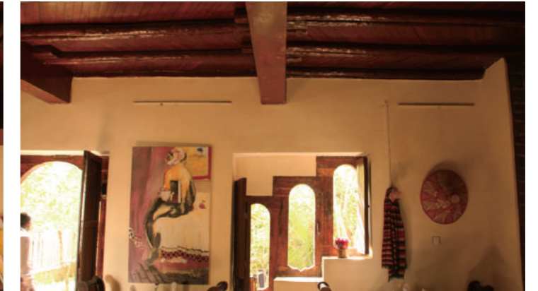
[9] Hidmo-inspired Timber Ceiling (Perhaps Beam is with RC member), photo by Shimizu, N., 2016
