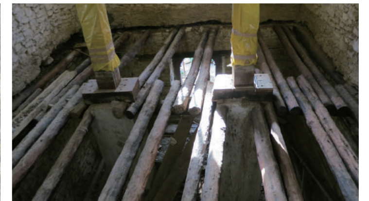
[14] During Restoration Work (Building-B), photo by Shimizu, N., 2012
