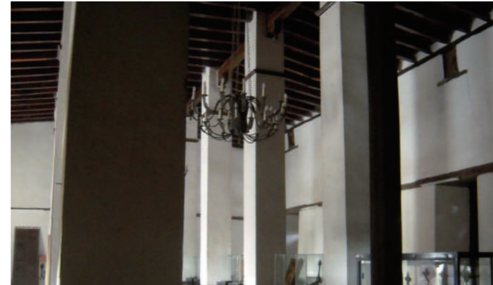
[8] Internal Appearance of Building-A (Ground Floor); Photo by Smidt, W., 2010
