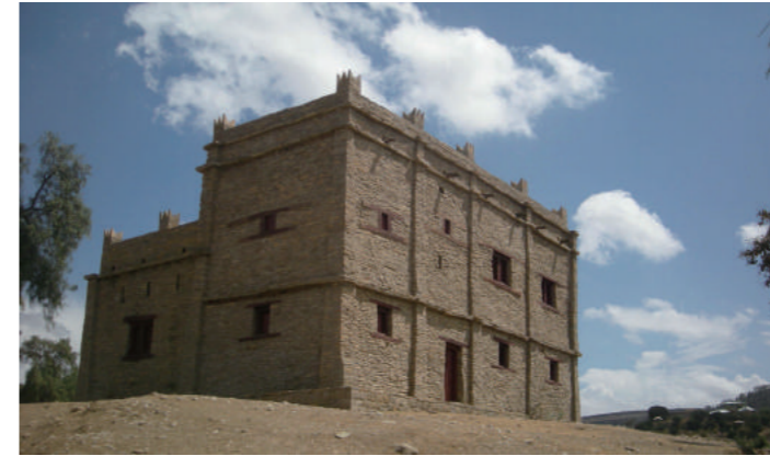
[6] External Appearance (from the Northwest), photo by Shimizu, N., 2011
