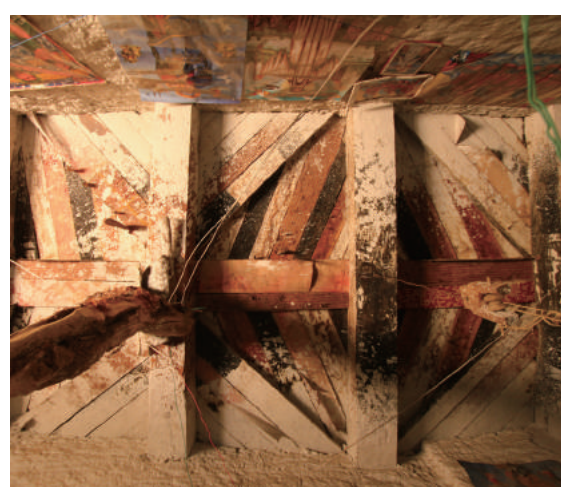
Fig.2-106 Simplified lantern ceiling in qiddist , Debre Sillasé Church, photo by author.
