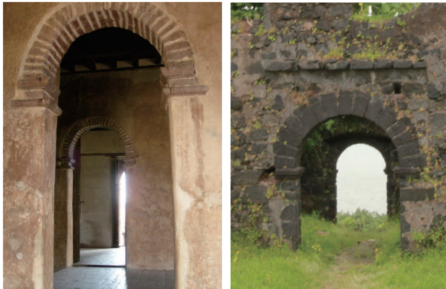
Fig.2-75 Arches found in Fasiledes Palace in Gonder (a) and Portuguese fort in Mumbai (b), photos by author.
