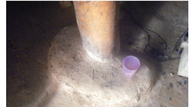
[6] Basement of a Pillar, photo by Sugawara, Y., 2010
