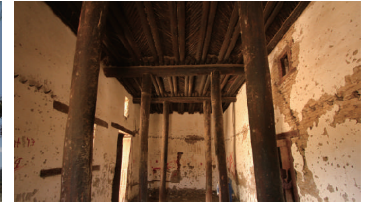
[7] Internal Appearance of Aderash (Ground Floor), photo by Shimizu, N., 2018
