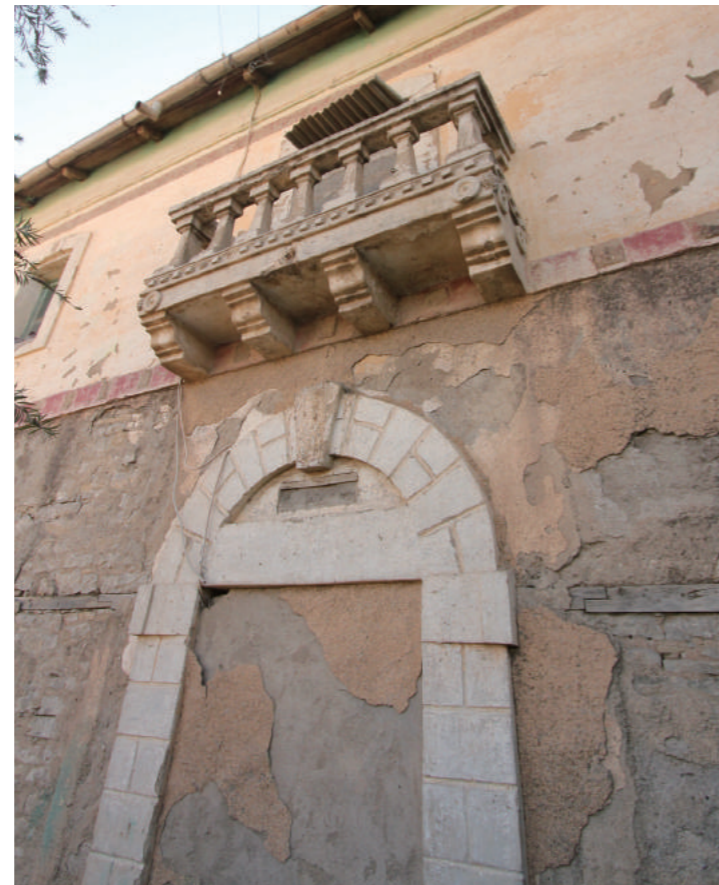
[4] Ornamental East Facade (Building-A), photo by Shimizu, N., 2018
