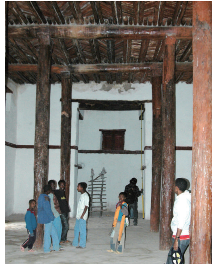
[6] Internal Appearance of Building-A, photo by Mano, Y., 2011
