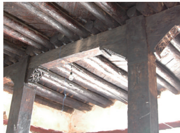
Fig.4-35 Timber ornamental pillars and ceiling, Former Residence of Emperor Yohannis IV (Building-B), photo by author.
