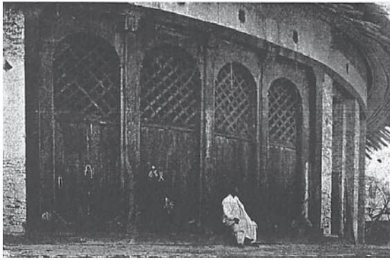
Fig.2-80 Four large timber ornamental openings on the west wall, Medhané 'Alem Church in 'Adwa, from Littmann et al. (1913).
