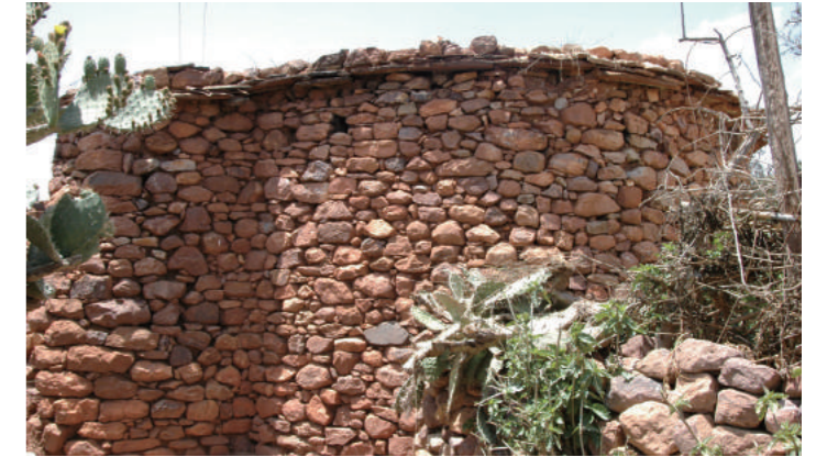
[2] External Appearance (from the Southeast), photo by Mano, Y., 2011
