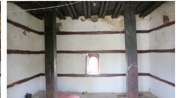
[7] Internal Appearance of Building-B (Upper Floor), photo by Shimizu, N., 2012
