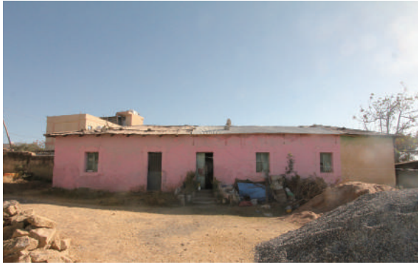
Fig.4-152 External appearance from the courtyard, Building-B of Old Hospital Quarter, photo by author.
