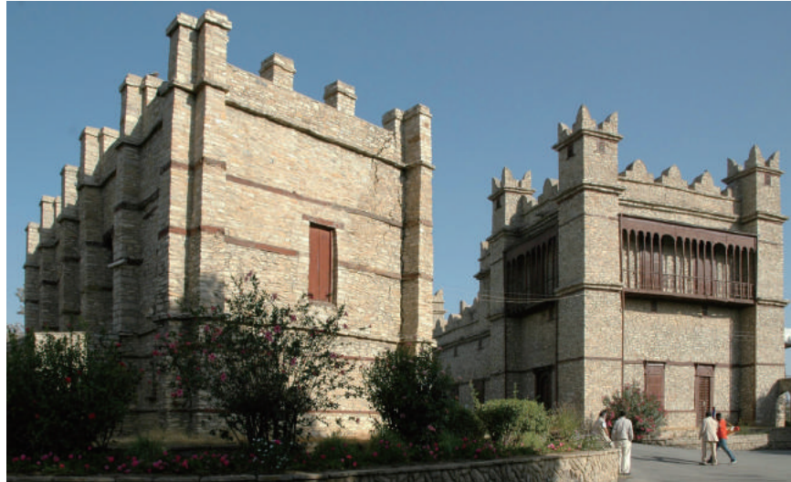
Fig.4-52 View of the buildings of Emperor Yohannis IV Palace (before restoration), collection of IPHC.
