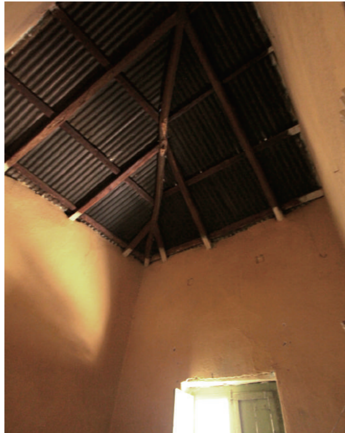
[5] A Southwest Room with Corrugated Metal Sheet Roof, photo by Shimizu, N., 2016
