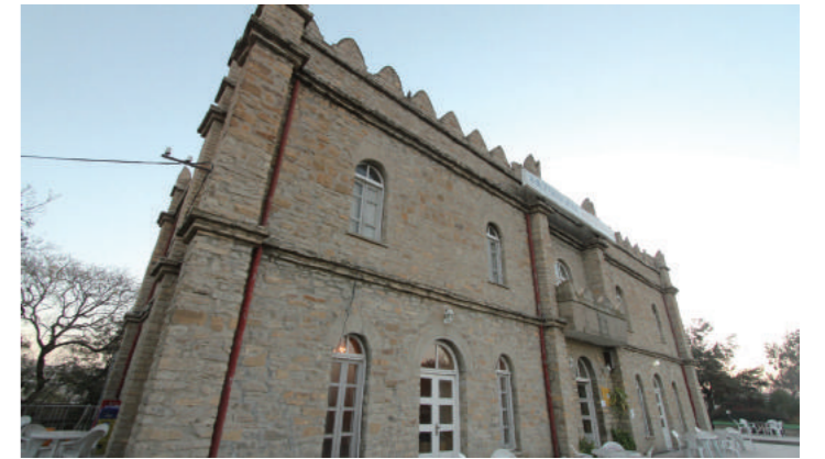
[6] External Appearance of Building-A (from the Northeast), photo by Shimizu, N., 2018
