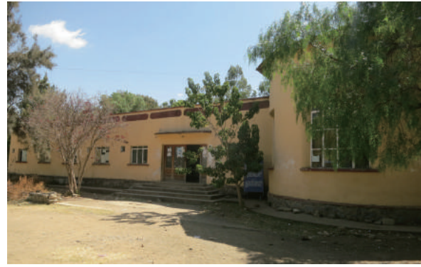
Fig.4-64 An example of a building in Kwiha erected in Italian occupation period, photo by author.
