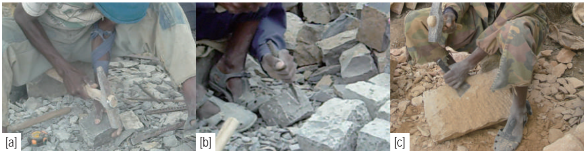
Fig.3-48 Workflow to shape a stone (a: Scraping a stone outline by martello ; b: Scraping stone surface by iskarbélo ; c: Smoothing a stone surface by t'efit'afa iskarbélo ), photo by author.
