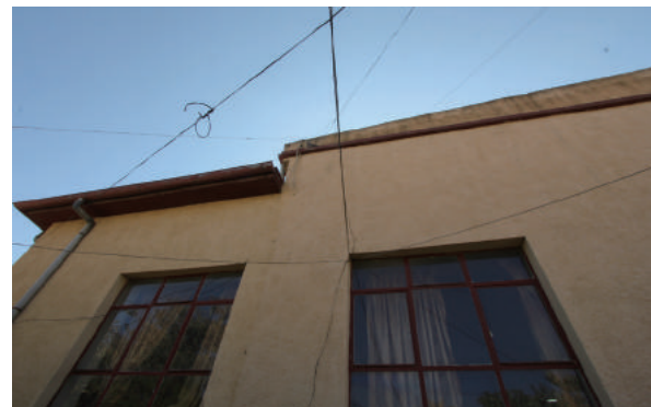
Fig.4-131 A wall of Italian Administrative Building, photo by author.
