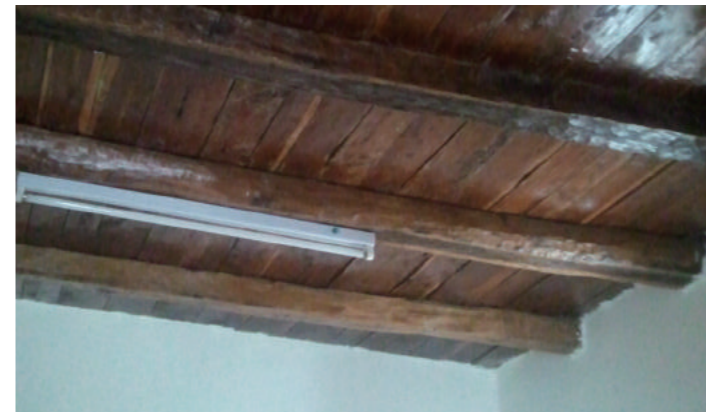
[6] Timber Ceiling of Ground Floor, photo by Shimizu, N., 2012
