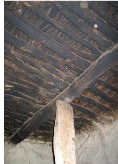
Fig.3-22 The ceiling with unshaped rugged natural woods, from Lyons (2007).
