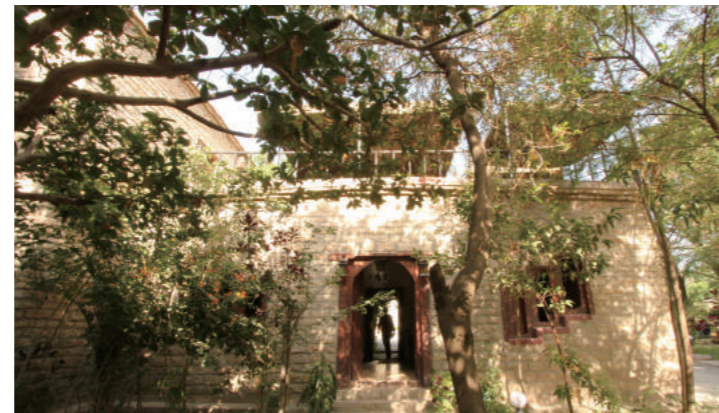
[3] External Appearance (from the Northwest), photo by Shimizu, N., 2016
