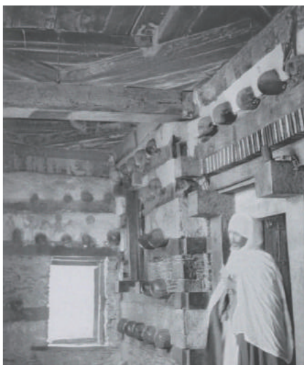
Fig.2-41 Lantern ceiling in anteroom, main church of Debre Dammo, from Phillipson (2009).
