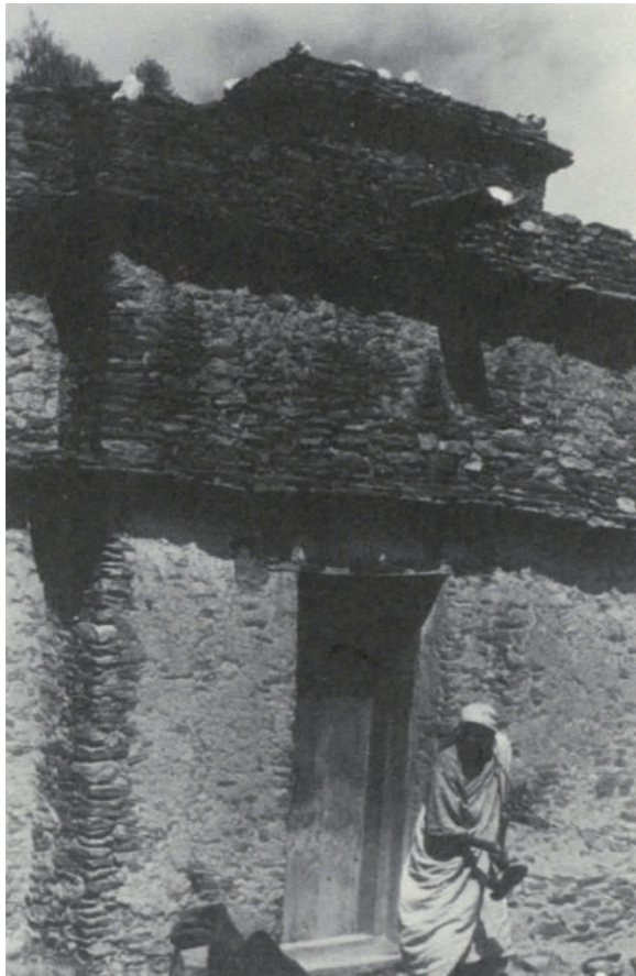
[2] External Appearance (from the South, 1970s), from Plant, R., 1973
