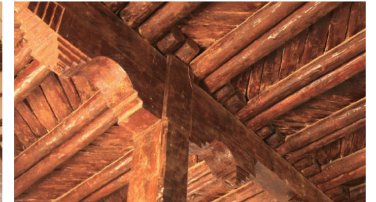
[11] A Timber Ornamental Pillar and Ceiling in a Room on the West Side in the Upper Floor (in Common with Hida), photo by Shimizu, N., 2018
