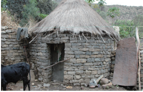
Fig.3-49 A circular masonry wall with stone pieces scraped in arc shape, photo by author .
