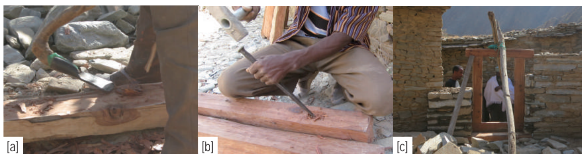
Fig.3-63 Workflow of wood processing (a: shaping a wooden surface; b: making a hole; c: embedding a door frame in the predetermined position); photo by author.
