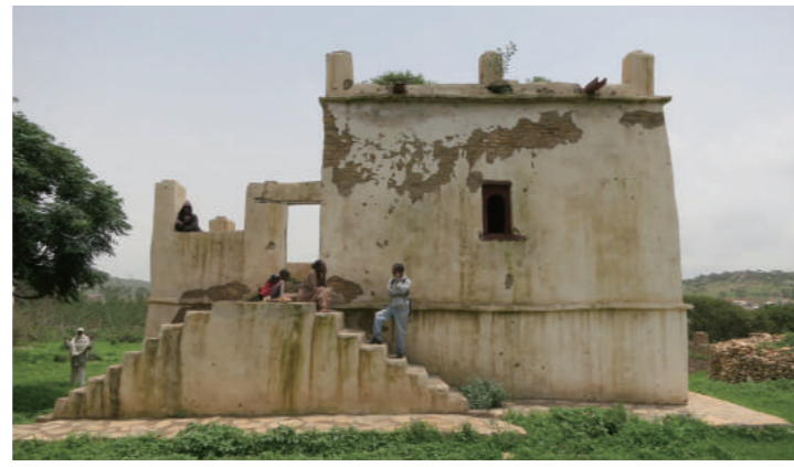
[3] External Appearance of Building-B approx. 1.5 Years after Plastering (from the South), photo by Shimizu, N., 2012
