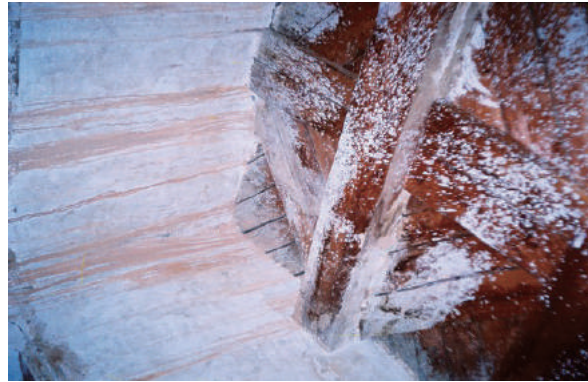
Fig.2-97 Simplified version of lantern roof applied in the old church of Asir Metira Monastery, photo by Mitik G. (taken before the removal of ceiling).
