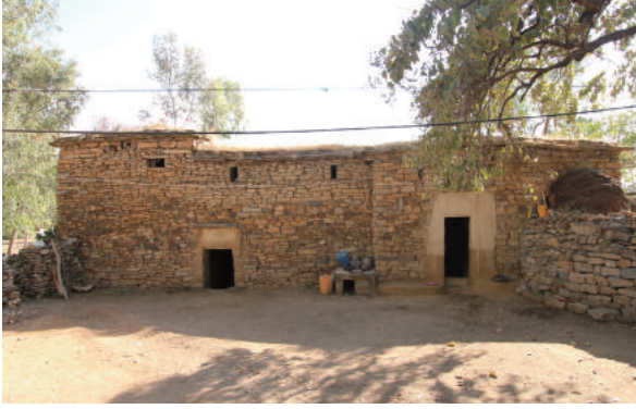
Fig.3-18 A door lower than body height (1022 mm; left building), photo by author.
