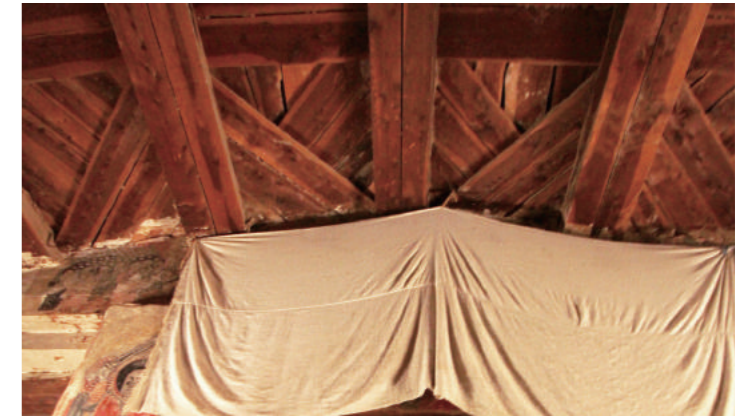
[7] Slightly Gabled Ceiling, photo by Shimizu, N., 2016
