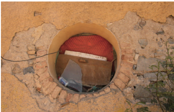
Fig.4-155 A circular window with brick frame, Building-C of Old Hospital Quarter, photo by author.
