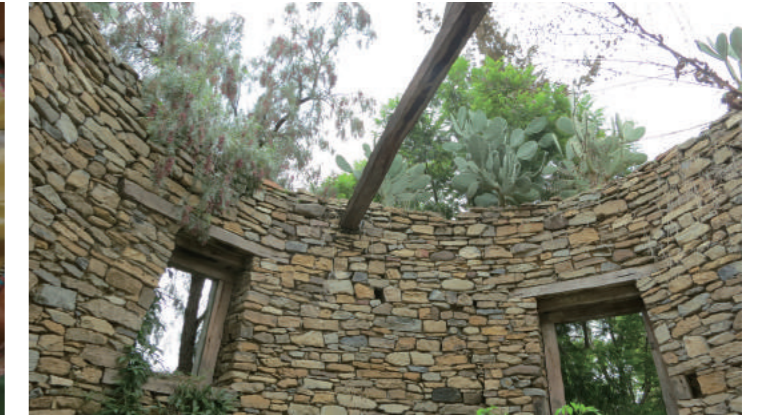
[7] Uncovered Roof with a Remaining Beam (Building-B), photo by Shimizu, N., 2012
