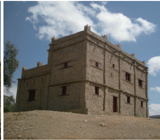
Fig.4-27 External appearance from the northwest, Ar'aya Castle, photo by author.
