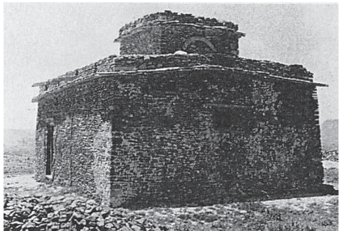
Fig.2-102 External appearance of "Debre Sillasé Church," from Juel-jensen et al. (1974).
