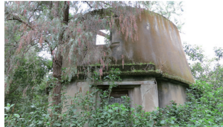
[3] External Appearance of Building-B (from the Southwest), photo by Shimizu, N., 2012
