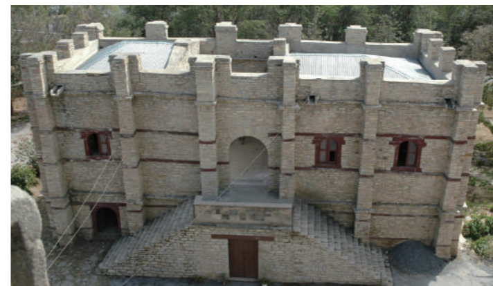
[13] External Appearance of Building-B (Shortly before the Restoration), Collection of IPHC
