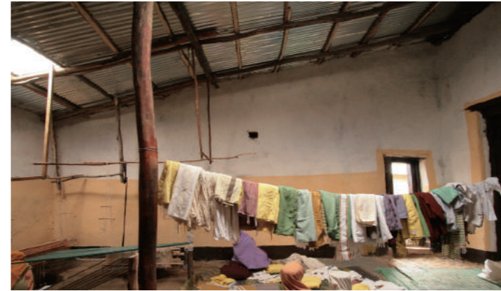
[19] Internal Appearance after Meqdes Wall Demolished, photo by Higuchi, R., 2010
