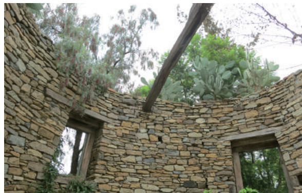
Fig.4-105 A beam, Building-B of Gugsa's Second House, photo by author.
