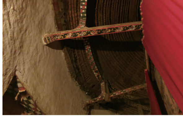
Fig.2-85 Beams, post and ceiling of Sillasé Church in Ch'eleqot, photo by author.
