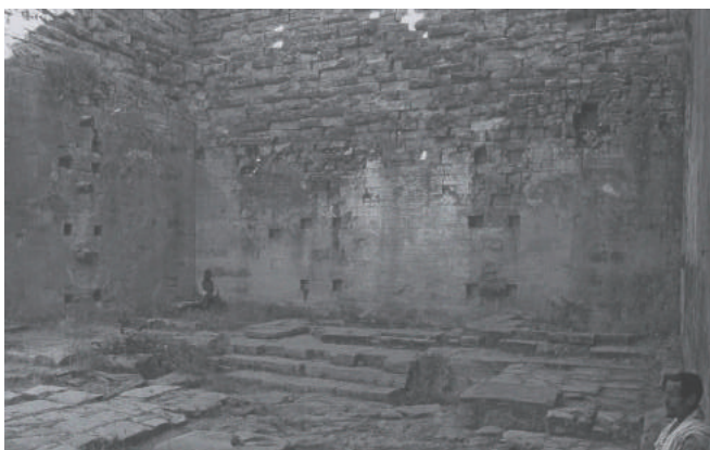
Fig.2-19 Mortises in the wall of Great Temple of Yeha, from Phillipson (2009).
