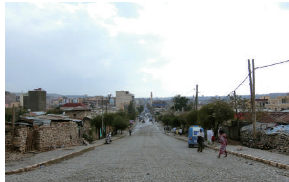
Fig.1-26 View from around the entrance of Maryam Church, photo by author.
