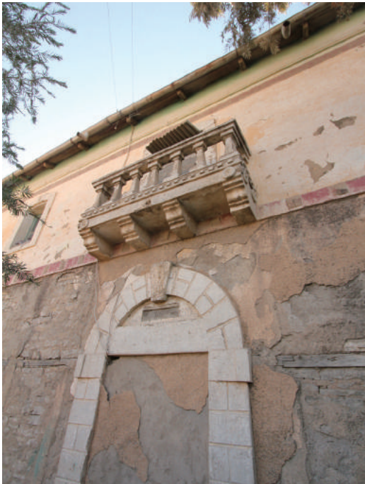
Fig.4-150 A wall of Building-A of Old Hospital Quarter, photo by author.
