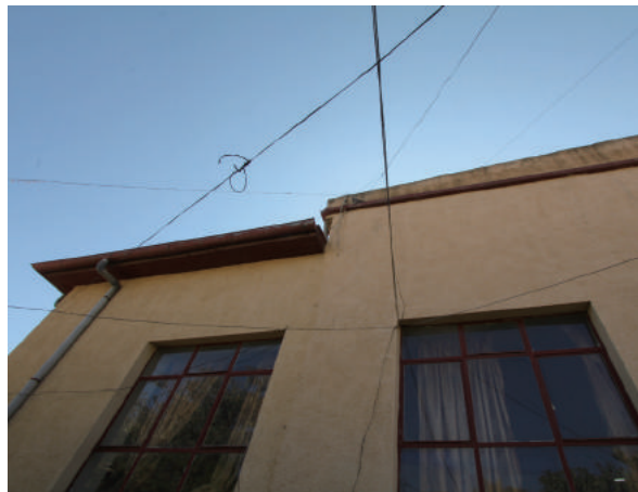
Fig.4-133 External appearance from the south, Italian Administrative Building, photo by author.
