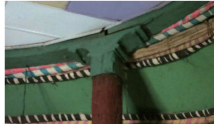
[8] Detail of a Timber Ornamental Pillar (Building-A), photo by Shimizu, N., 2012
