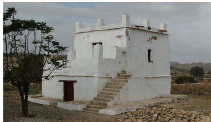
[5] External Appearance of Building-B (from the Southwest), photo by Mano, Y., 2011
