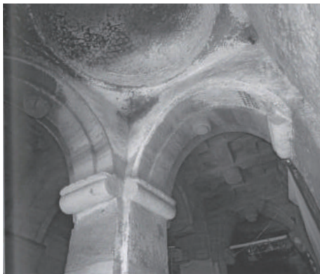
Fig.2-66 Arches with bracket capitals in anteroom, Maryam Wigro, from Phillipson (2009).
