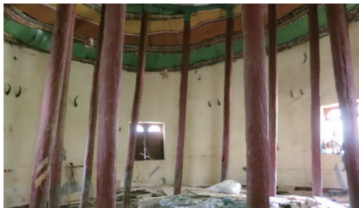
[4] Internal Appearance of Building-A, photo by Shimizu, N., 2012
