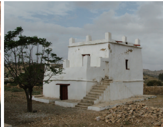
Fig.4-33 External appearance from the southwest, Former Residence of Emperor Yohannis IV (Building-B), photo by Mano, Y.
