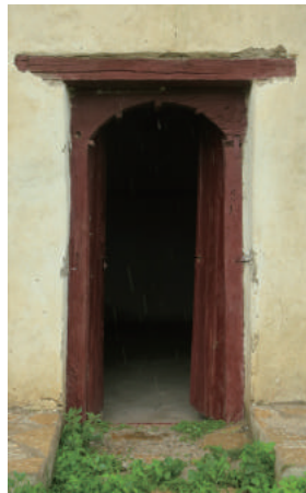
Fig.4-40 A timber arched opening with bead-planks, photo by author.
