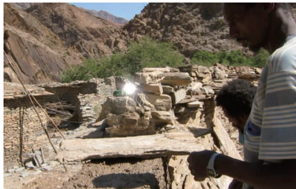
Fig.3-21 Thinner stones with a large surface area that cover the top of wall, photo by author.
