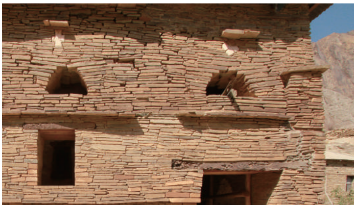
Fig.2-130 Corbel arches in the east wall, Debre Garzén of Gunde Gundé, photo by author.
