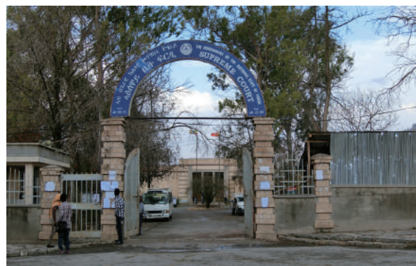
Fig.4-80 Italian Administrative Building (presently Supreme Court Building) placed in an iconic position, photo by author.
