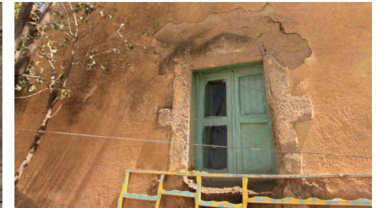
[6] An Opening in the West Side (Building-A), photo by Shimizu, N., 2018
