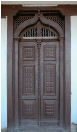
Fig.4-51 Timber ornamental door with ogee arch applied in the main building of Emperor Yohannis IV Palace, collection of IPHC.
