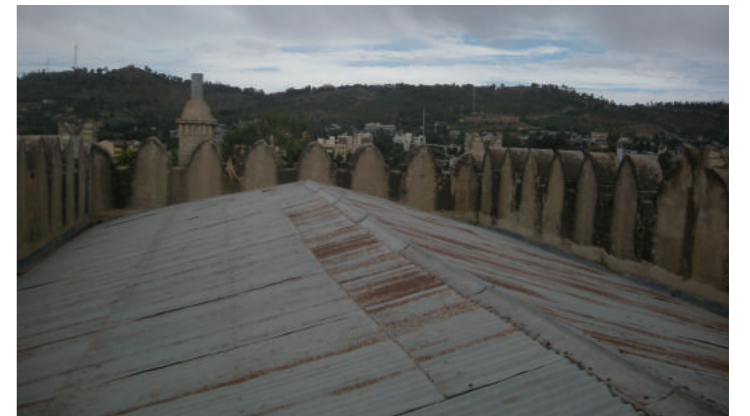
[10] Corrugated Metal Sheet Covering Building-A, Photo by Shimizu, N., 2011
