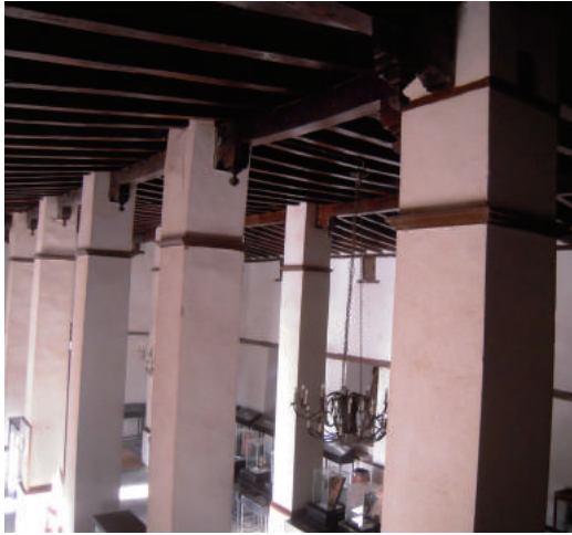
Fig.4-56 Masonry pillars with timber ornament and timber ceiling, main building of Emperor Yohannis IV Palace, photo by Smidt, W.
