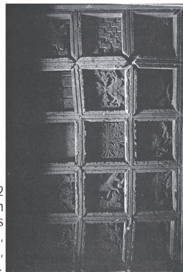
Fig.2-42 Ceiling consisting of coffered construction of square wooden panels with relief carving in vestibule, main church of Debre Dammo, from Littmann et al. (1913).
