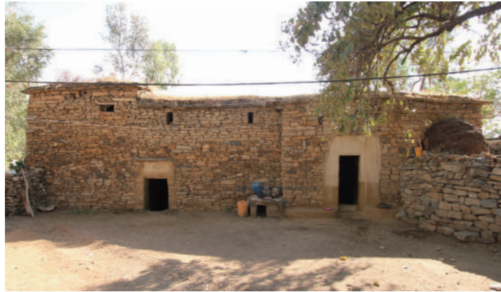
[1] External Appearance (from the North), photo by Shimizu, N., 2015
