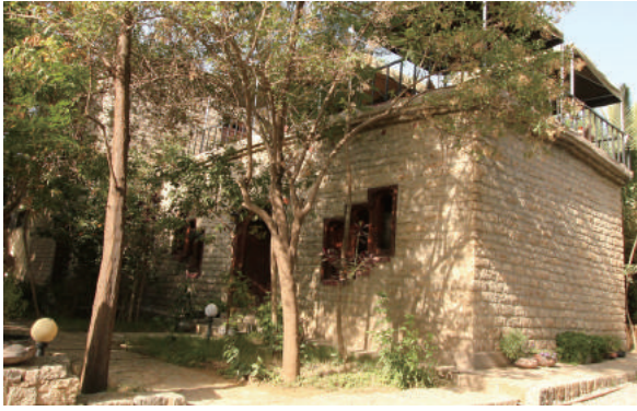
Fig.4-188 External appearance of Mengesha's Second House, photo by author .
