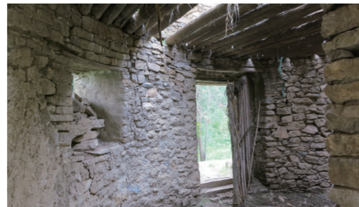
[5] Internal Appearance of Building-A, photo by Shimizu, N., 2012
