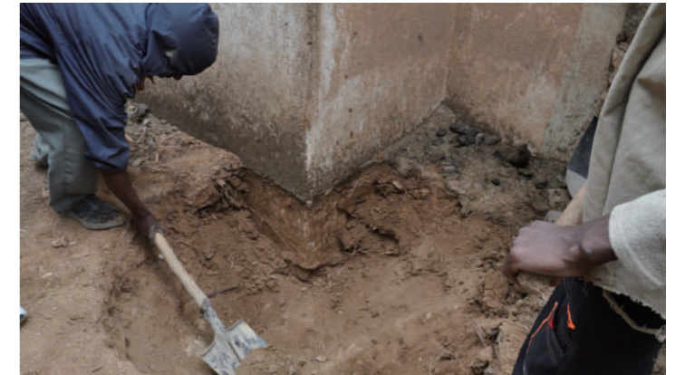
[24] Building Foundation, photo by Miyake, R., 2011
