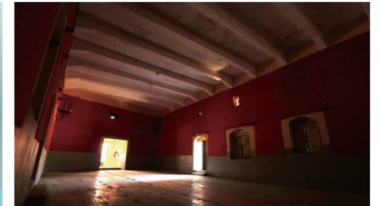
[9] A Hall in the A-Part (Reinforced Concrete Roof is not Original), photo by Shimizu, N., 2016
