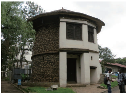
Fig.2-12 External appearance of "Tigré Chief's House" relocated to EiABC in Addis Abeba, photo by author.
