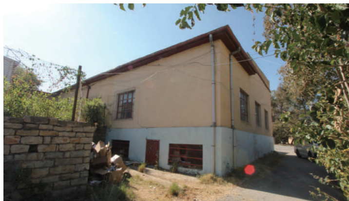
[4] External Appearance (from the North), photo by Shimizu, N., 2015
