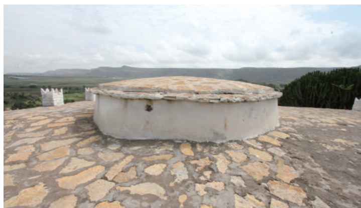
[4] Roof over the Area of Qiddíst, photo by Shimizu, N., 2014
