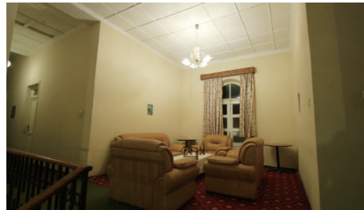
[9] Lobby with Panel Ceiling in the Upper Floor of Building-A (Perhaps the Work in the Time of Renovation), Photo by Shimizu, N., 2018
