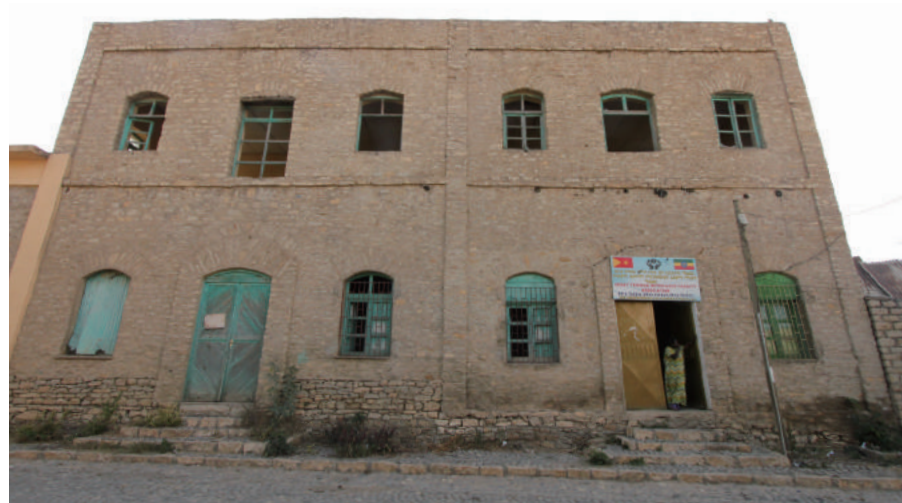
Fig.4-118 External appearance of Liquor Factory from the street, photo by author.
