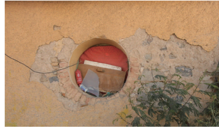
[20] A Circular Window with Brick Rim and Stone Masonry Wall (Building-C), photo by Shimizu, N., 2018
