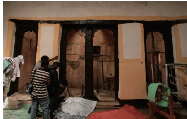
Fig.2-94 Timber screen between qiddist and qiné mahlét, old church of Asir Metira Monastery, photo by Higuchi, R.
