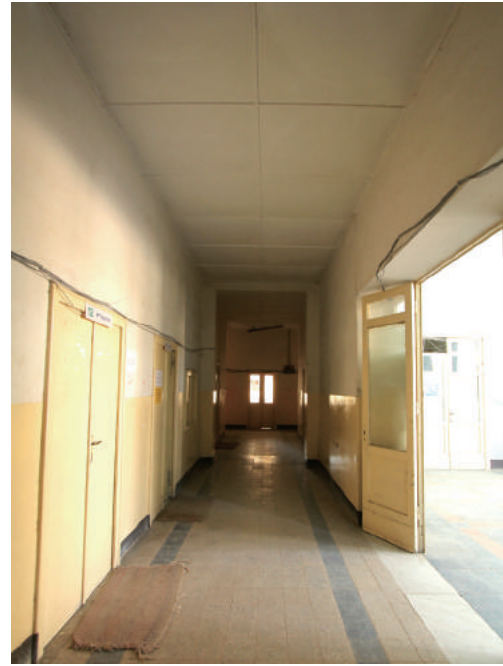
Fig.4-135 A corridor with wooden panels, Italian Administrative Building, photo by author.
