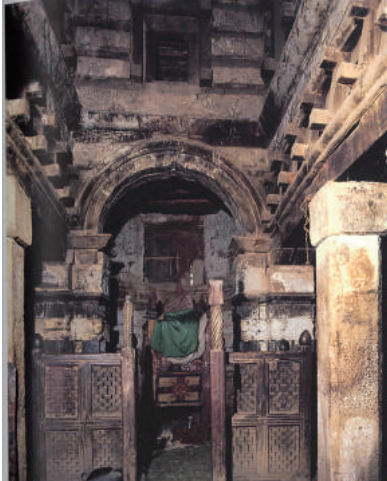
Fig.2-51 Internal appearance of nave, Zeréma Giyorgis, from Lepage et al. (2005) .
