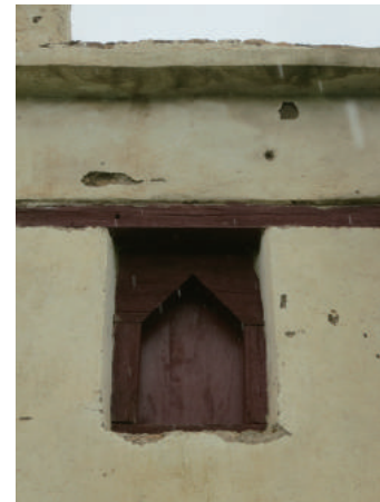
Fig.4-41 A triangular shaped opening found in Building-A, photo by author.
