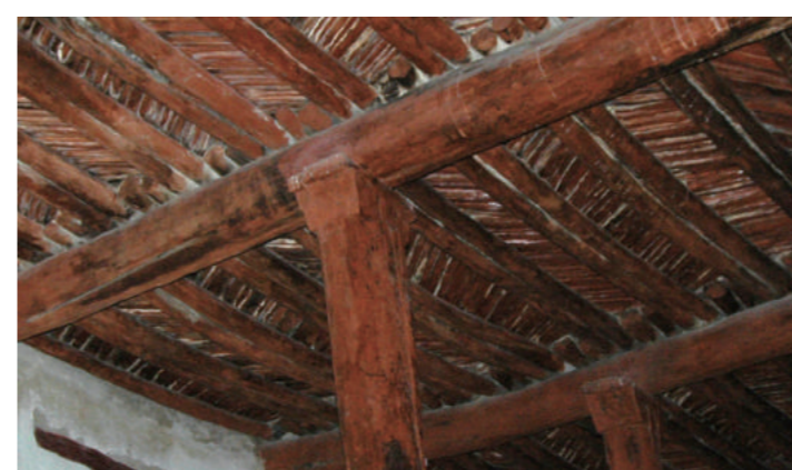
[9] Timber Ornamental Pillars and Ceiling of Building-A (in Common with Hidmo), photo by Mano, Y., 2011
