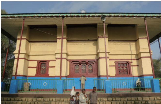
Fig.2-133 External appearance from the west, Abune Gebre Menfes Qïddus Church, photo by author .
