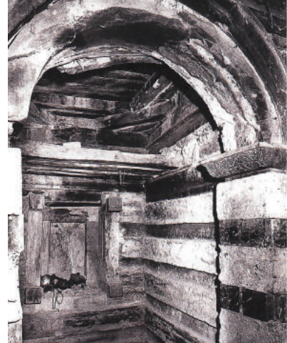
Fig.2-53 Northern transept with lantern ceiling (now demolished), Zeréma Giyorgis, from Lepage et al. (2005) .
