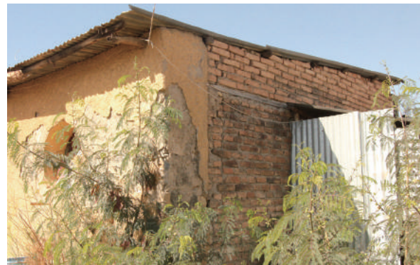
Fig.4-156 Brick-used northside wall, Building-C of Old Hospital Quarter, photo by author.
