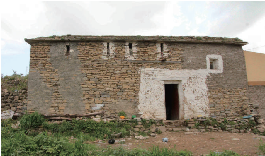
Fig.2-10 External appearance of hidmo , photo by author.
