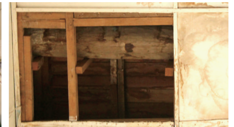
[13] The Slab Structure Composed by Timber Members (Photo Taken from the Ground Floor, B-Part), photo by Shimizu, N., 2016
