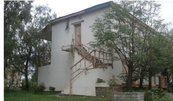
[3] External Appearance (from the Northwest), photo by Shimizu, N., 2012
