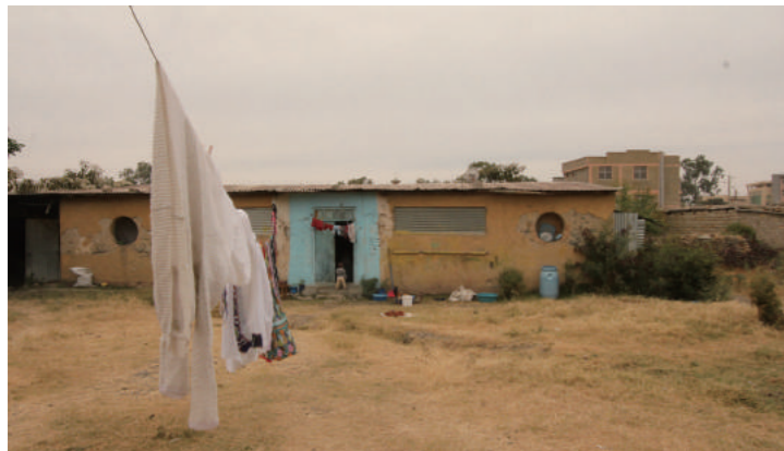
[18] External Appearance of Building-C (from the East), photo by Shimizu, N., 2016
