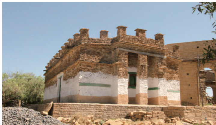
[4] External Appearance (from the Northwest), photo by Shimizu, N., 2016
