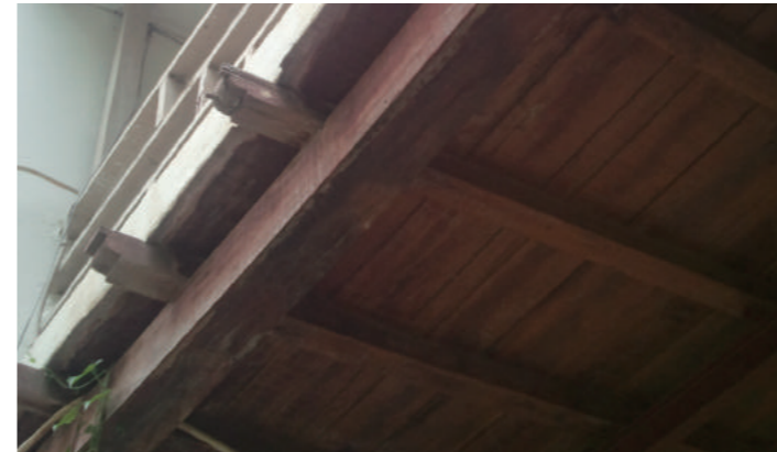
[4] Floor of Veranda, photo by Shimizu, N., 2012
