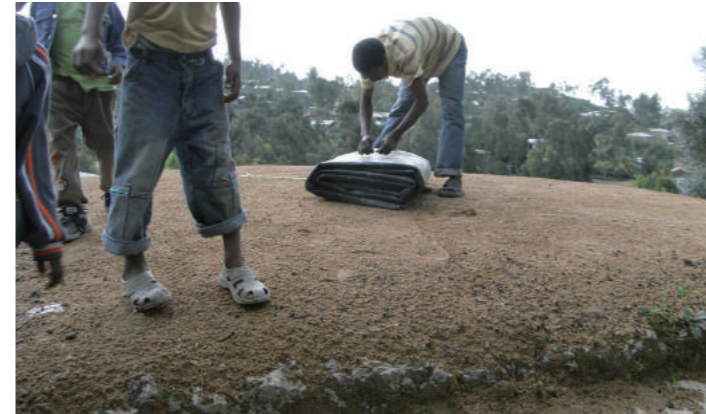
[3] Detail of Hidmo Roof, photo by Mano, Y., 2010
