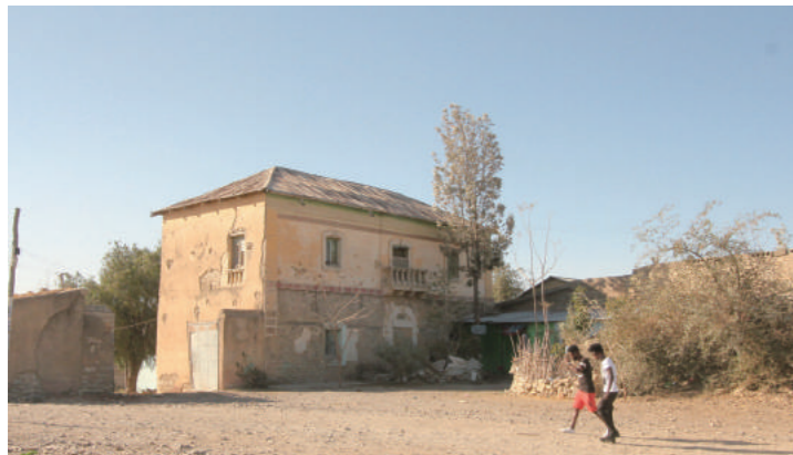
[2] External Appearance of Building-A (from the Southeast), photo by Shimizu, N., 2018
