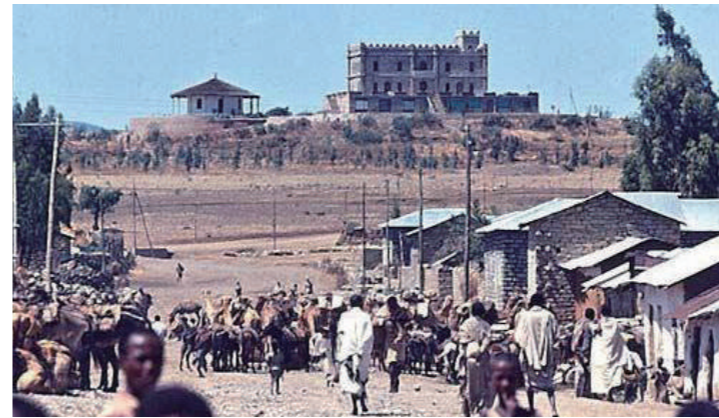
[5] During Renovation Work (perhaps ca. 1950s), source unknown
