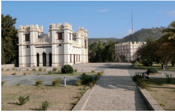
Fig.4-47 View of the buildings of Emperor Yohannis IV Palace in Mekelle (after restoration), photo by author.
