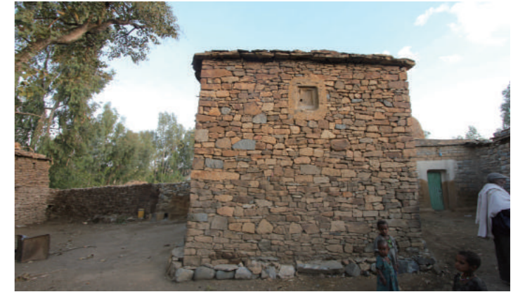
[2] External Appearance (from the North), photo by Shimizu, N., 2015
