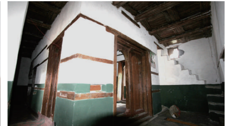
[7] Internal Appearance of Qiné Mahlét and Corridor, photo by Shimizu, N., 2014
