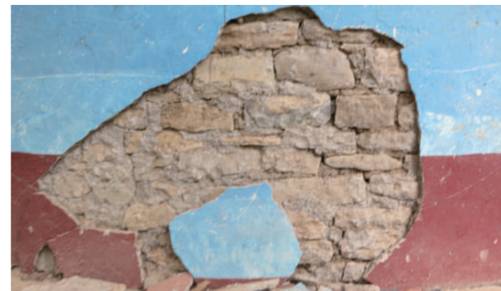
[12] Original Masonry Wall of Building-A, photo by Shimizu, N., 2012
