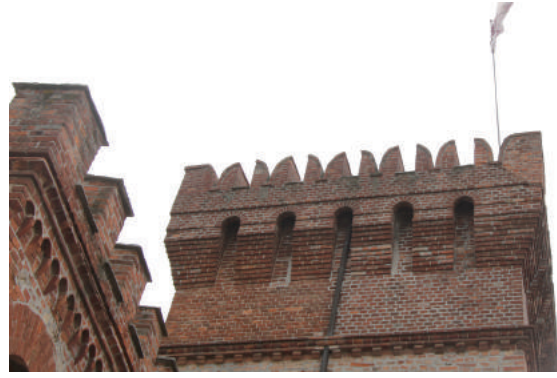
Fig.4-53 Parapets found in the castle located in northern Italy, of which design is similar with the main building of Emperor Yohannis IV Palace, photo by author.
