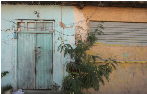
Fig.4-157 A horizontally long window installed in Building-C, Old Hospital Quarter, photo by author.
