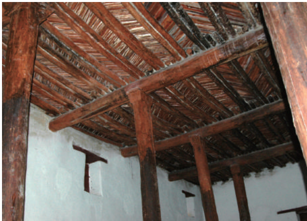
Fig.4-32 Timber ornamental pillars and ceiling, Former Residence of Emperor Yohannis IV (Building-A), photo by Mano, Y.
