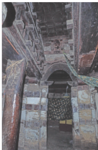
Fig.2-49 Internal appearance of nave with flat paneled ceiling, Qirqos Agobo, from Phillipson (2009).
