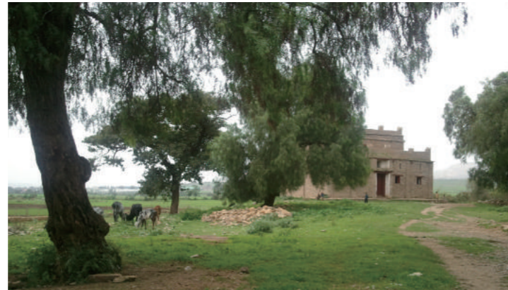
[3] Approach from the Southeast, photo by Shimizu, N., 2018
