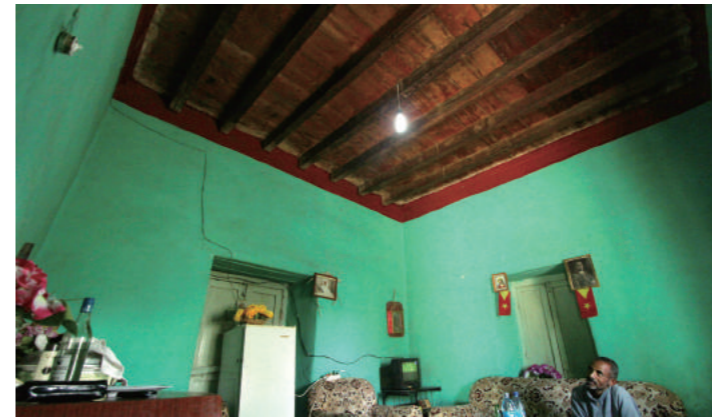
[5] A Ground Floor Room with Timber Ceiling, photo by Shimizu, N., 2016
