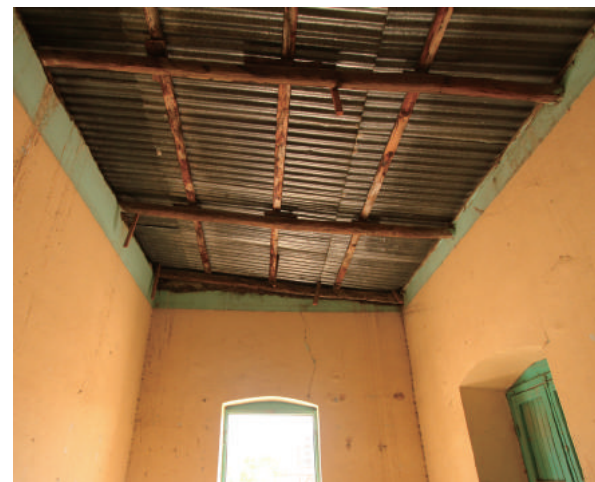
Fig.4-116 Roof structure exposed by ceiling unfastened, photo by author.
