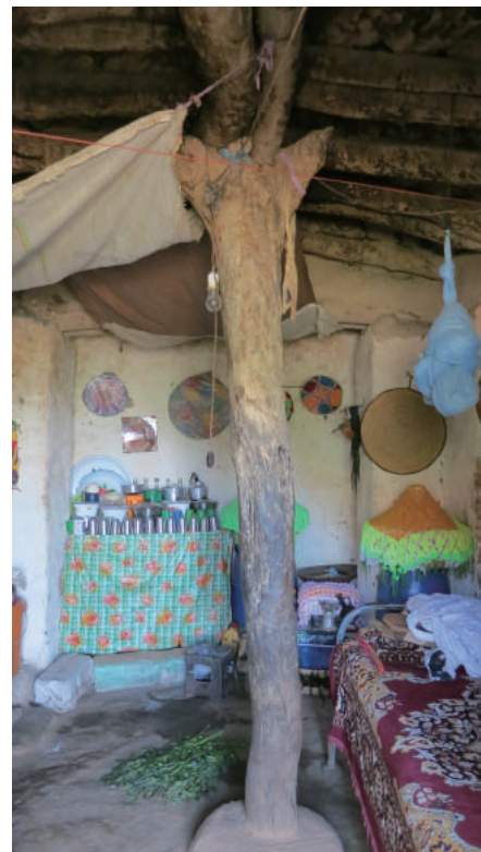
Fig.3-35 Internal appearance of hidmo house in Témben, photo by author.
