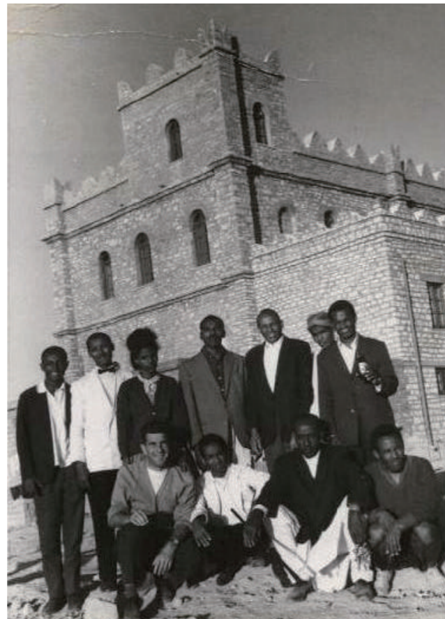
[4] At the Time of Renovation (ca. 1960; Right Part of the Building Extended), source unknown
