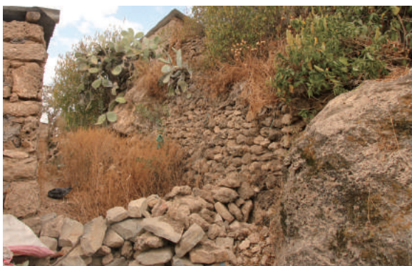
Fig.1-34 Stone piles applied in the gap of parcels in Īnda Mesqel, photo by author .
