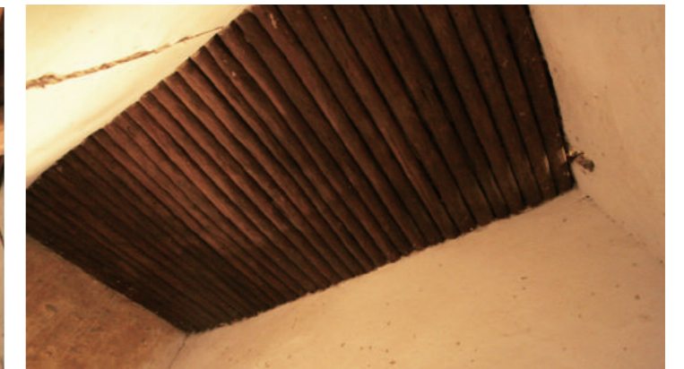
[13] Simpler Wooden Ceiling, photo by Shimizu, N., 2018
