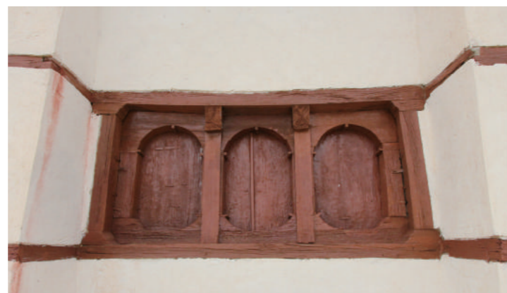
[5] A Tripartite Window in the West Side, photo by Shimizu, N., 2014
