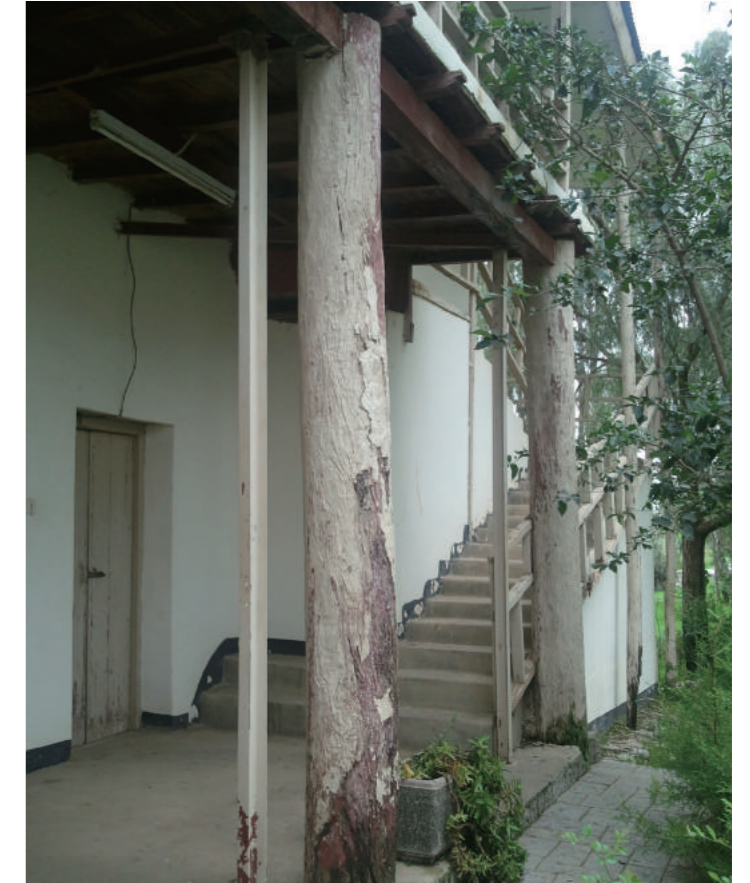
[5] Space under the Veranda, photo by Shimizu, N., 2012
