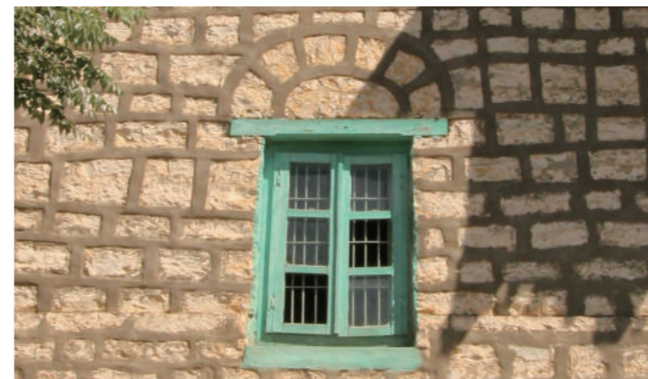
[9] An Opening in the West Side, photo by Shimizu, N., 2016
