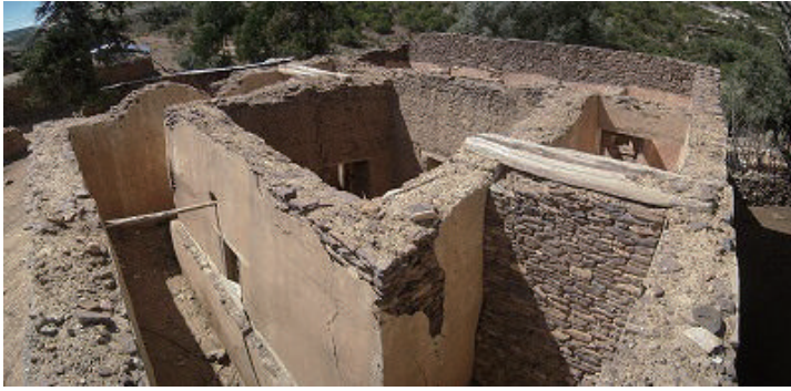
Fig.2-91 A top-down view from the northeast, old church of Asir Metira Monastery, photo by Miyake, R. (taken before the demolition of meqdes).
