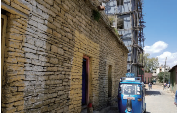
Fig.4-198 A hidmo roofed building next to a mid-rise building, photo by author .
