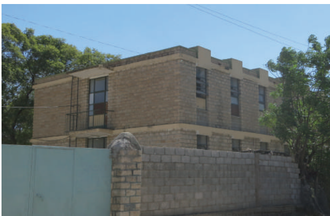
Fig.4-181 An example of RC structure building with stone masonry wall, photo by author.
