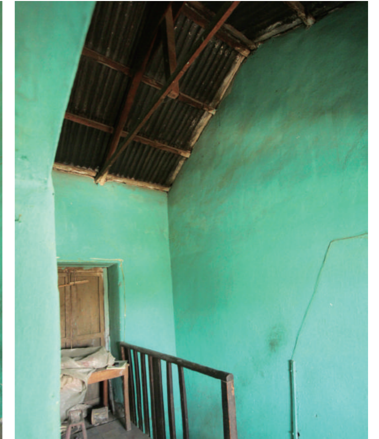
[8] A Stair Room in the Upper Floor, photo by Shimizu, N., 2016
