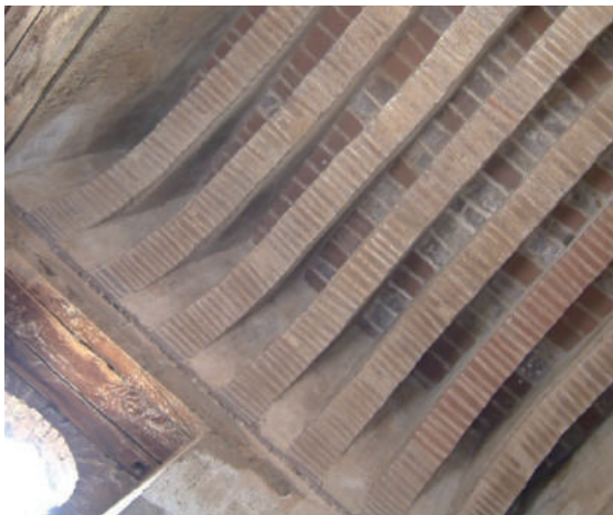
Fig.2-76 Transverse arches found in Iyasu I Palace in Gonder, from Shitara (2008).
