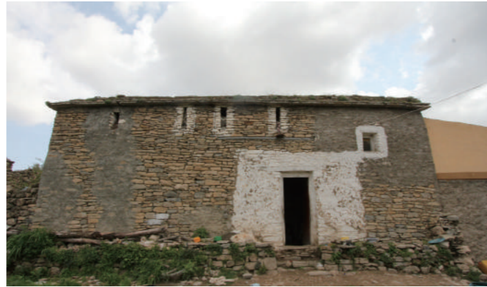
[2] External Appearance (from the North), photo by Shimizu, N., 2014
