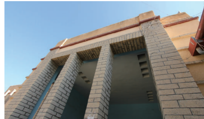
[6] An Entrance Porch, photo by Shimizu, N., 2015
