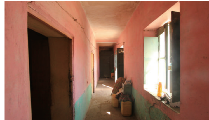
[26] Internal Appearance of Corridor (Building-D), photo by Shimizu, N., 2018
