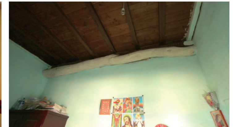
[9] Internal Appearance of a Ground Floor Room on the North Side (Building-A), with Timber Beams and Ceiling, photo by Shimizu, N., 2018
