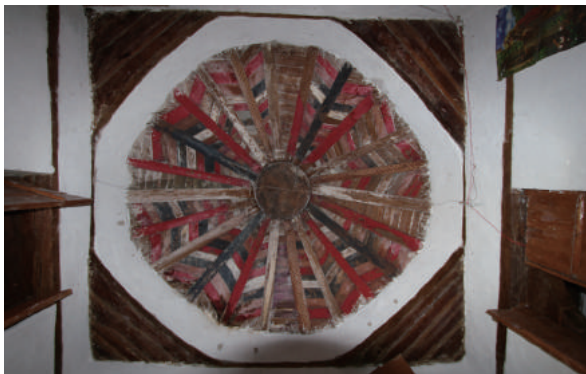
Fig.2-117 Timber dome installed in qiddist , Mika'el Church in Feleg Da'iro, photo by author.
