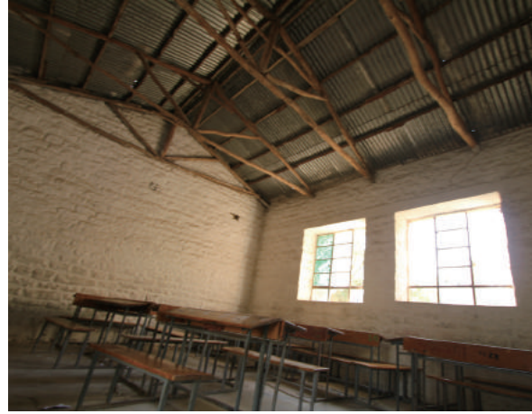
Fig.4-139 Roof structure exposed by ceiling unfastened, a School for Italians, photo by author.
