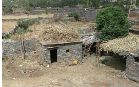
Fig.3-6 A flat roof placing a sheaf of straw, photo by author.
