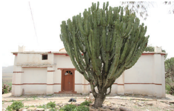
Fig.2-118 External appearance from the south, Mika'el Church in Feleg Da'iro, photo by author.
