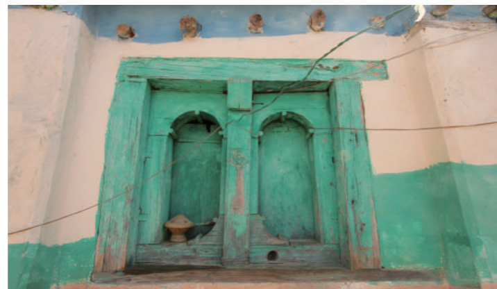
[5] A Timber Ornamental Window, photo by Shimizu, N., 2018
