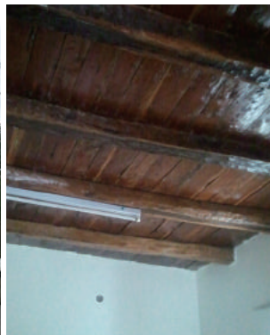
Fig.4-94 Ceiling of ground floor, Siyyum's Second House, photo by author.
