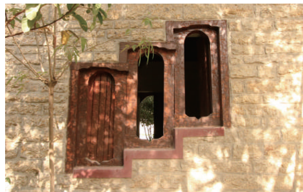
Fig.4-190 Window arrangement in tiers, Mengesha's Second House, photo by author .
