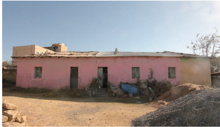
[12] External Appearance of Building-B (from the North), photo by Shimizu, N., 2018
