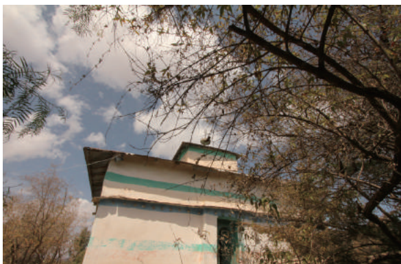
Fig.2-107 External appearance from the east, Debre Sillasé Church, photo by author .
