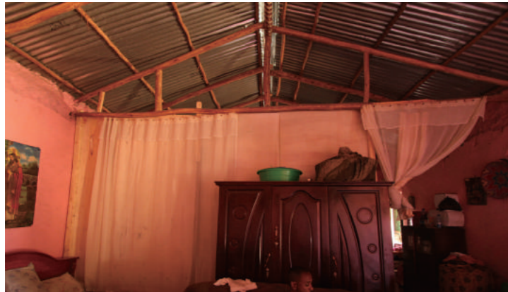
[16] Internal Appearance of Building-B after Reinforcement, photo by Shimizu, N., 2018
