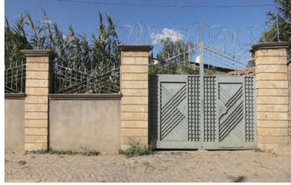
Fig.3-50 An outdoor wall enclosing a parcel made from stone pieces with smoothed surface, photo by author .
