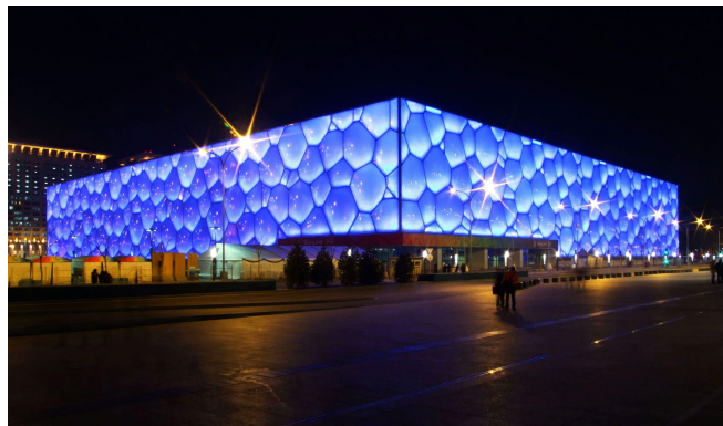
FIGURE 1.5: An example of computational design, the olympic pool for Beijing 2008 games. Designed by PTW Architects, CSCEC,CCDI and Arup
