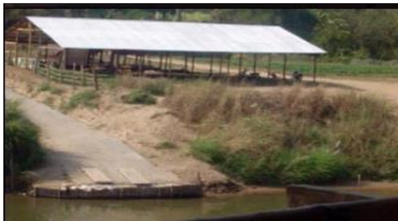
Figure 5.7: Warehouse and concrete ferry dock at gate number 12 along the Thai-Myanmar border
