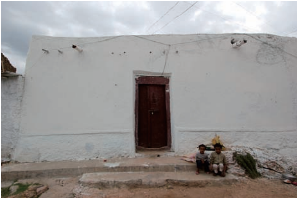
Fig. 5-28 Main façade of old Harari house built 600 years ago (left)
