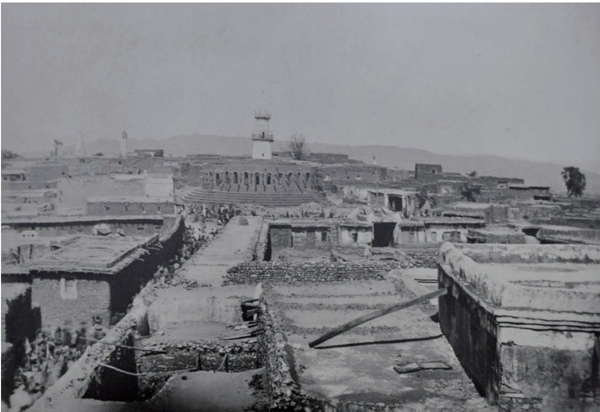
Fig. 1-61 Medhane Alem Church under construction, from the rooftop, 1888-1889
