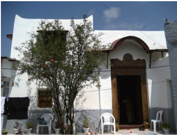
Fig. 5-4 Façade of Wober house
