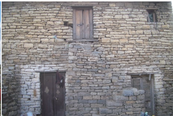
Fig. 4-32 Photo of Blata Assefa Abay before demolition from the back, 2009 (right)
