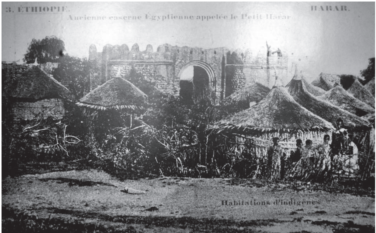
Fig. 1-63 Thatched roof houses ( gambisa ) of Harar, 1888-1889
