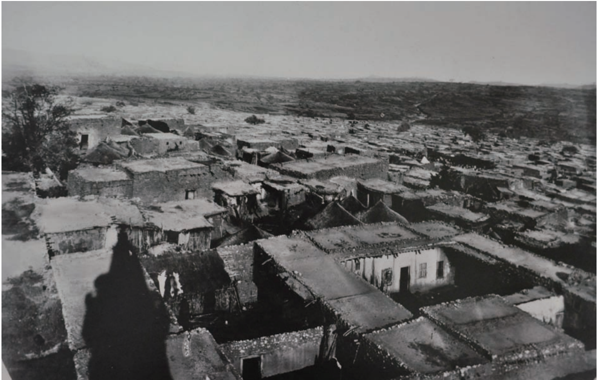
Fig. 1-62 Flat roof houses of Harar, 1888-1889
