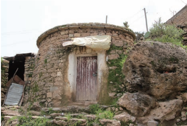
Fig. 4-17 Round house type building in Enda Meskel area
