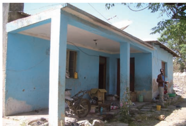
Fig. 4-19 Villa type constructed in reinforced concrete
