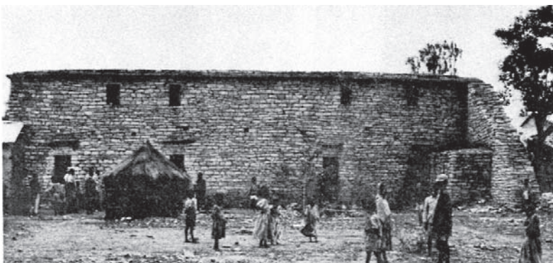
Fig. 4-15 Photo of a double story rowhouse type building
