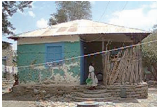
Fig. 4-37 Former residence of Nigsti Desta, Italian villa type house made of chikka
