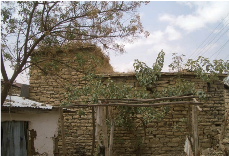
Fig. 4-7 Lumped Tri-parted House in study area
