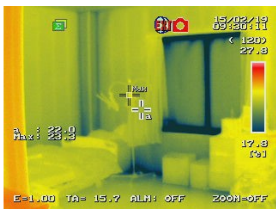
Figure 3.7 Thermal image photograph in facility 25
