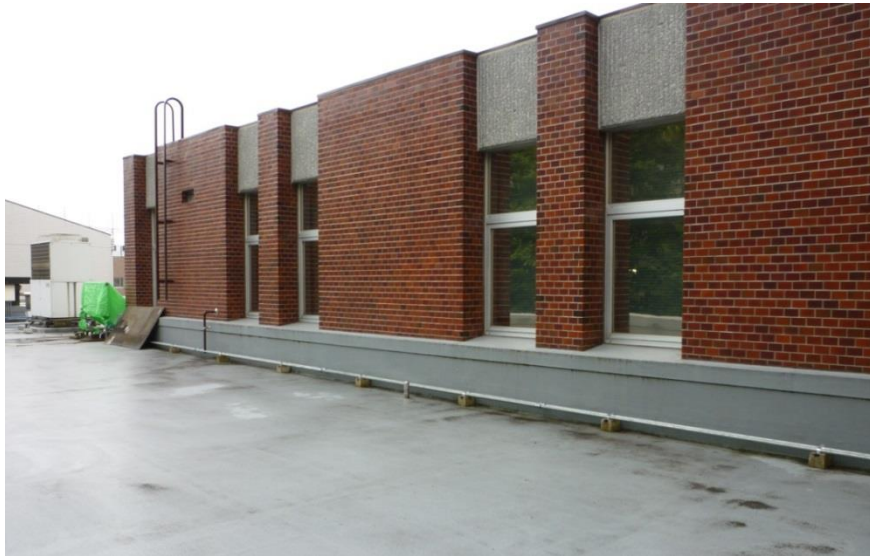
Fig. 13 Experiment site at Yagami Campus, Keio University in Yokohama, Japan
