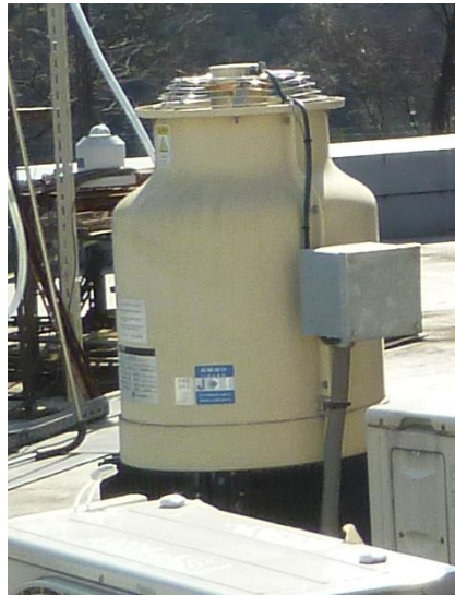
Fig. 29 Cooling tower
