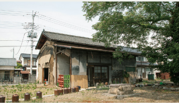
Old sake brewery before renovation
