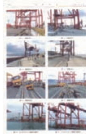
Fig. 1:Port Damage in Kobe 1995
