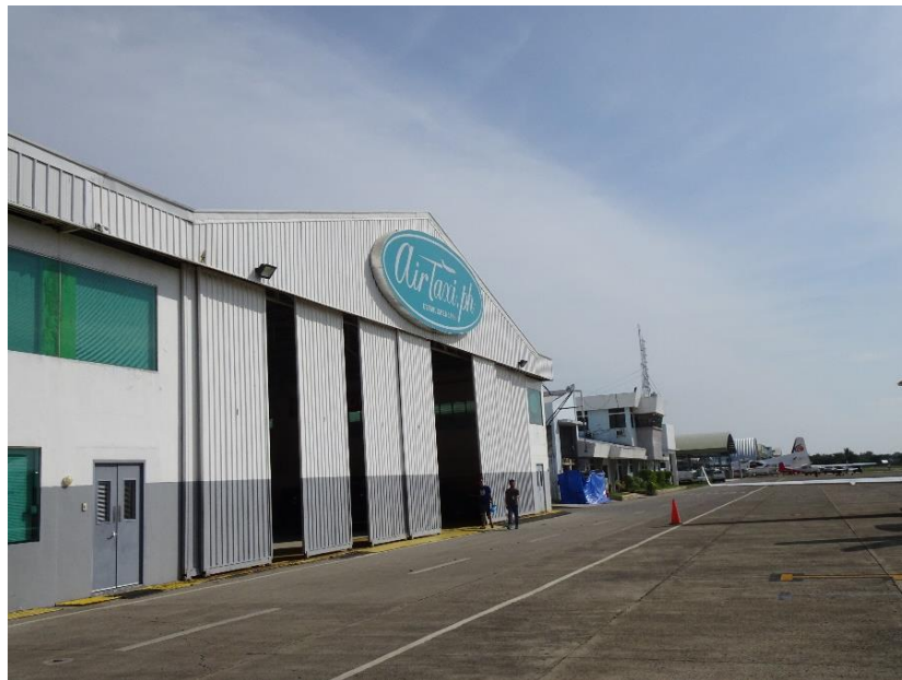
Figure 5: AirTaxi PH Cebu hangar in Mactan Island [Photo from author]
