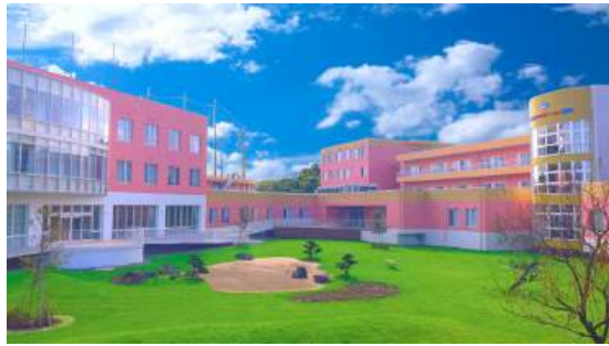
Figure 5.1 Yachiyo Rehabilitation Hospital, a local medical facility that is involved in occupational therapy methods
