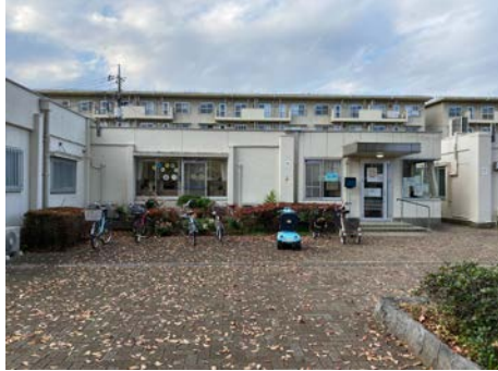
(a) Hokkori building
