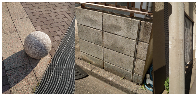
Figure 2.1 Concrete in Different Shapes
