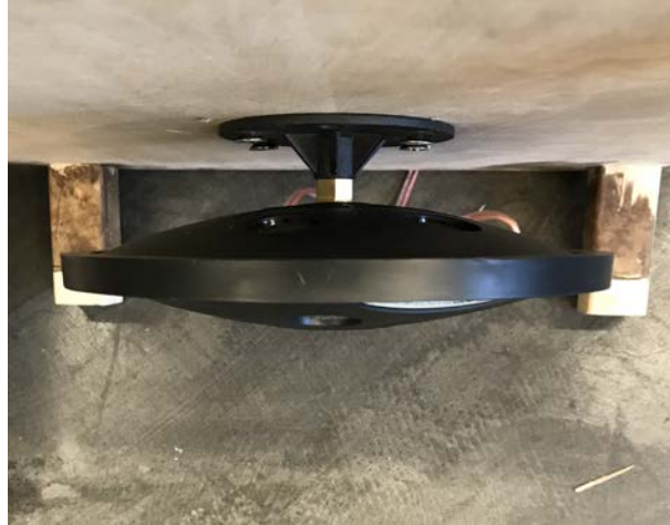
Figure 3.4: Placement of Transducer
