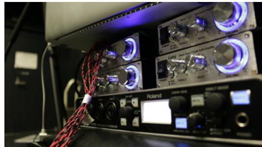
Figure 3.31: Amplifiers and Audio Interface
