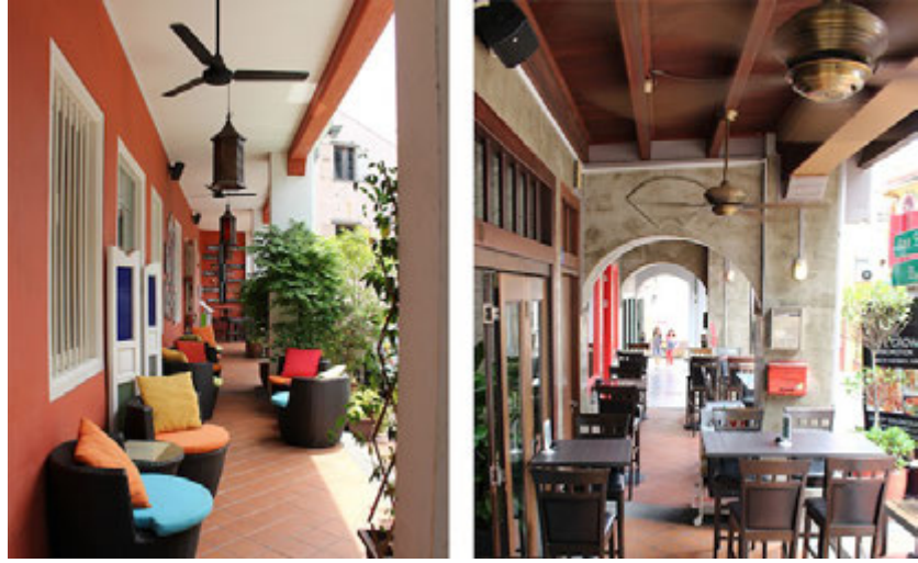
Figure 1.5: Ceiling fans installed in arcade-style buildings
