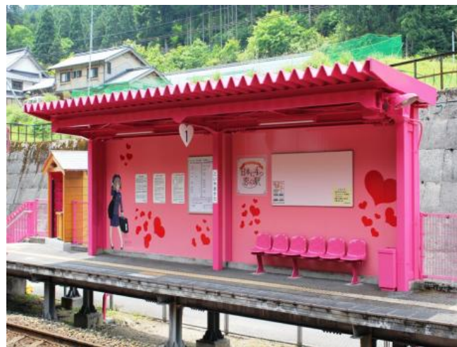
Figure3.4: Love Station Project – Koi Yamagata Station. [30]
