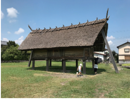
Image 19.7: Late Yayoi period raised floor building at Toro Site 登呂遺跡 (34.956720, 138.408346). (23 August 2020)
