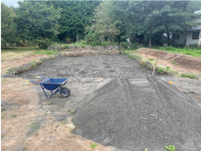
Figure 4: Suwahara site after excavation. The site was protected with sandbags placed in trenches and pits, covered in two blue tarps, and filled with sand. (26 September 2021)
