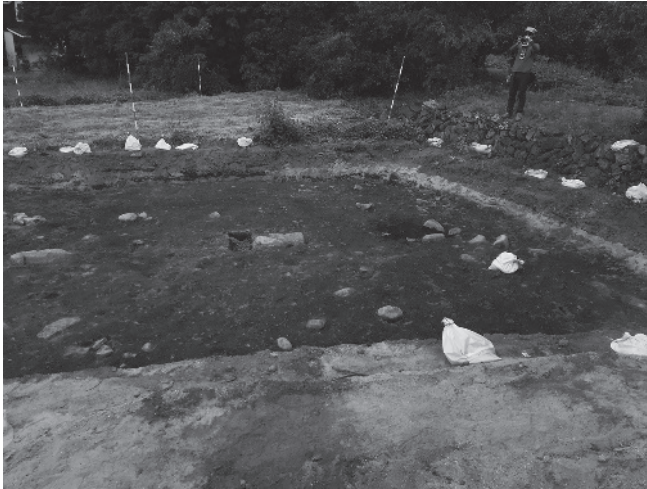
Figure 9: Suwahara site at the end of excavation work. (20 September 2019)
