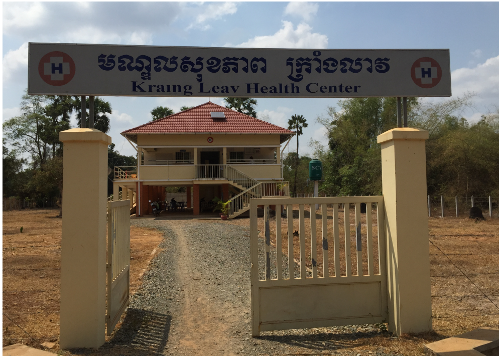
Figure 6 Provincial health center visited for fieldwork
