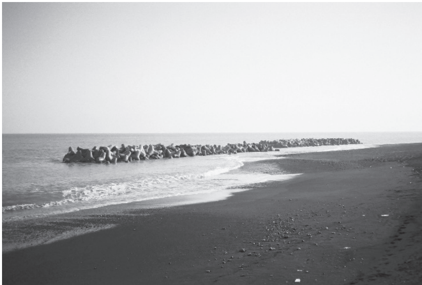
Fig. 9 Offshore breakwaters of Miho Coast
